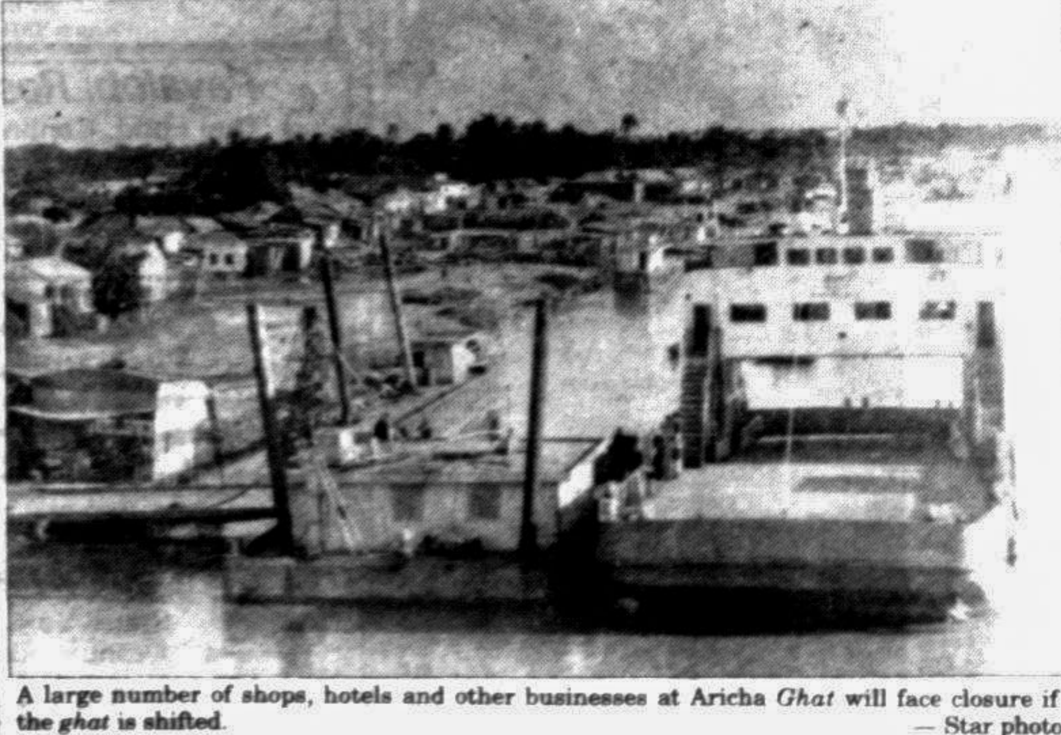
A large number of shops, hotels and other businesses at Aricha Ghat will face closure if the ghat is shifted. — Star photo
