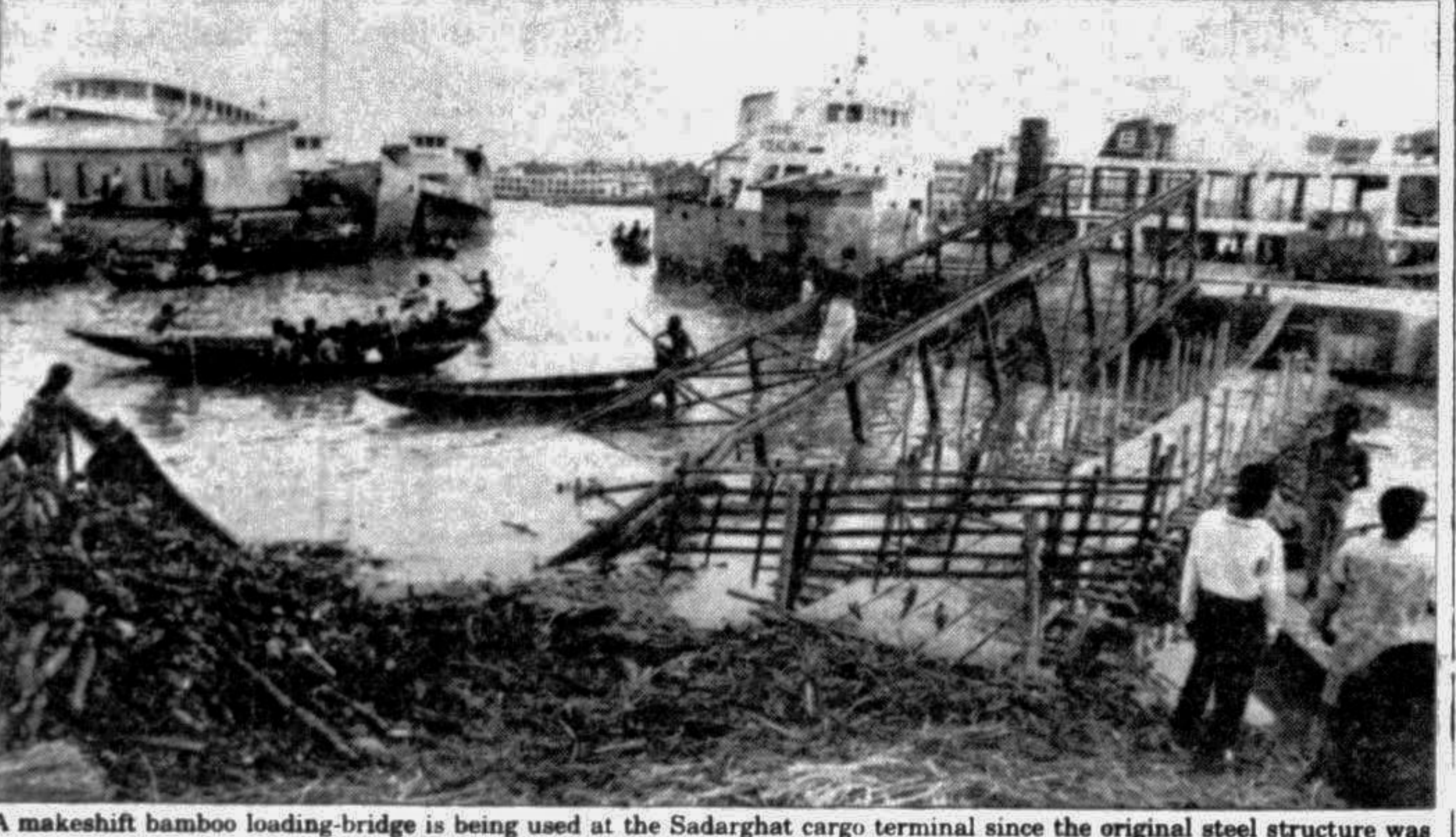
A makeshift bamboo loading-bridge is being used at the Sadarghat cargo terminal since the original steel structure was damaged quite sometime ago. —Star photo by Anisur Rahman
