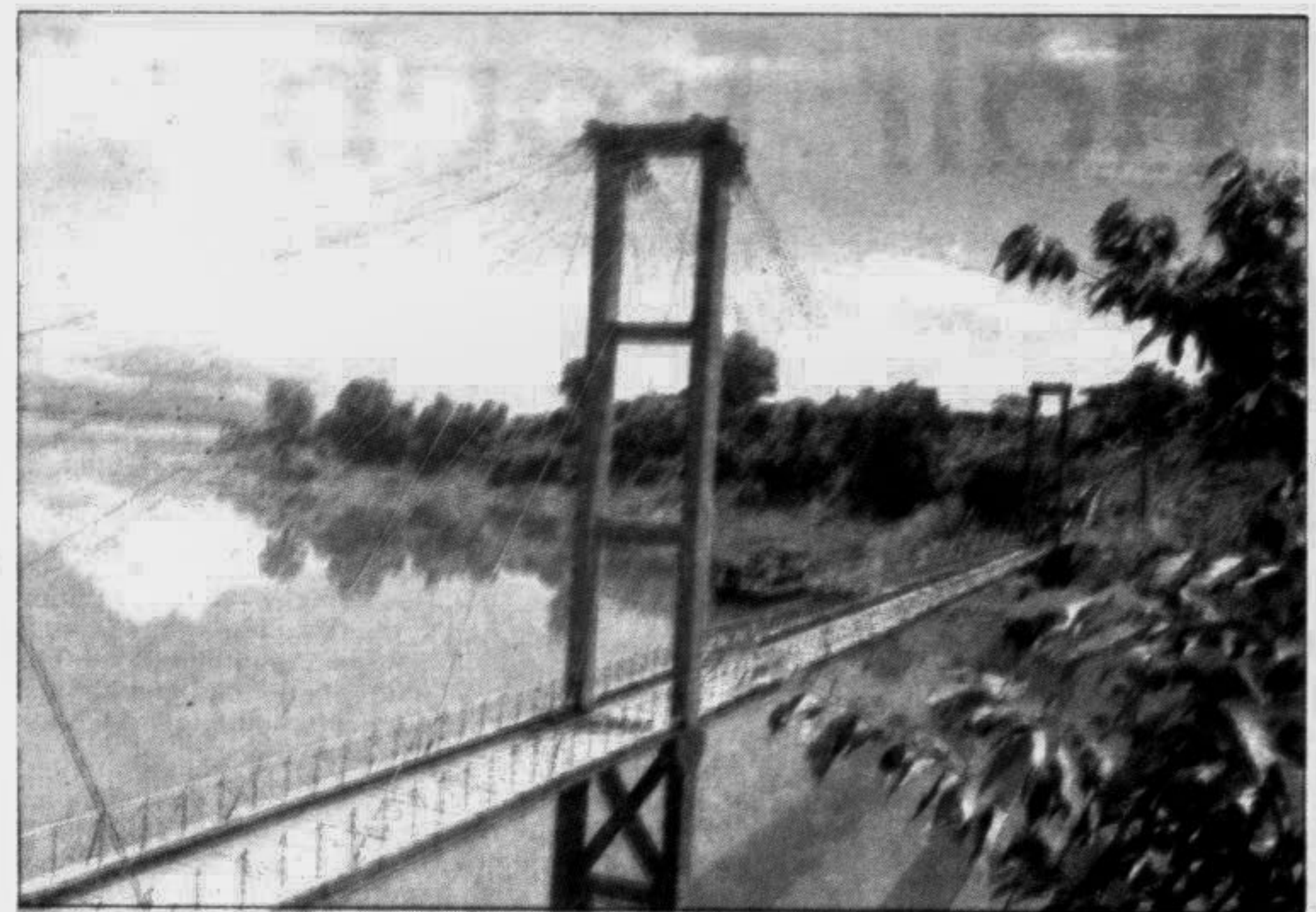
Walking along the suspension bridge is a rewarding experience
