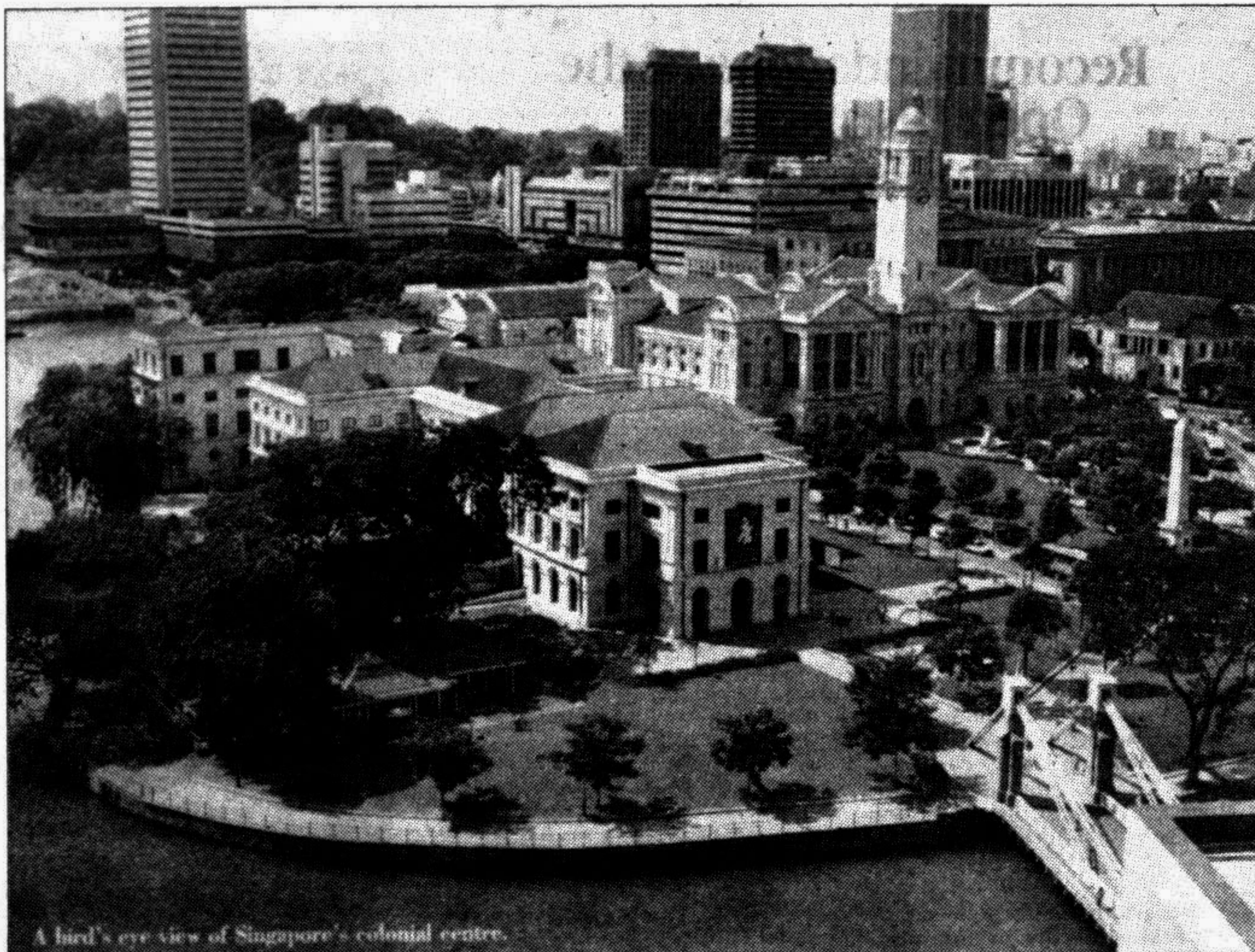
A bird's eye view of Singapore's colonial centre.
