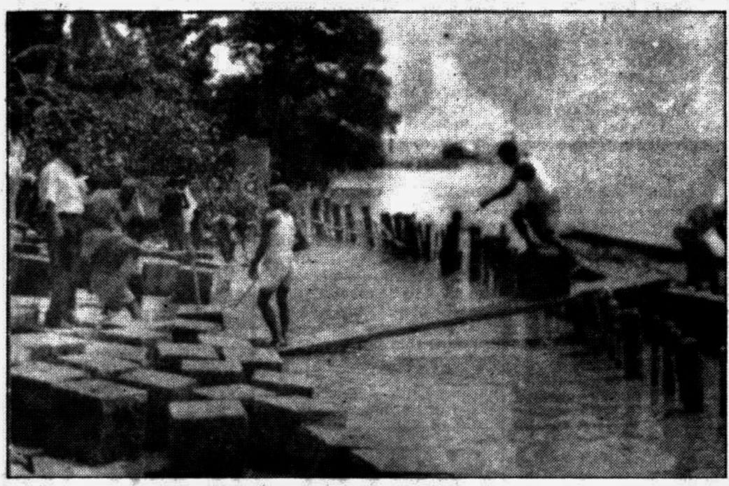
again threatened by erosion CHANDPUR: Blocks of concrete are being dumped by BWDB in a bid to thwart erosion of — Star photo
