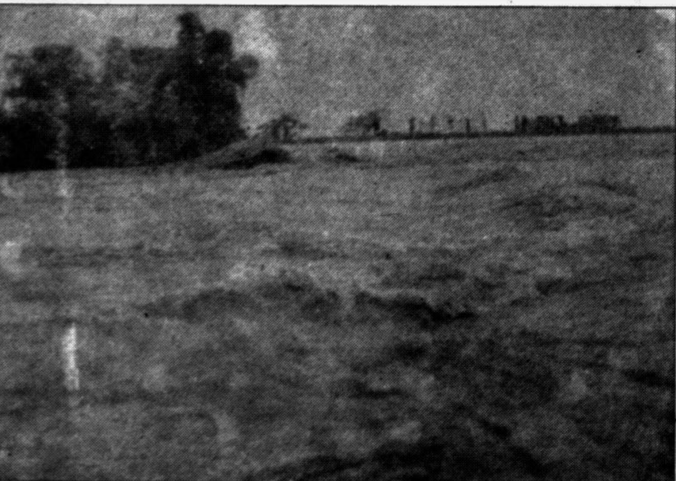
SYLHET: Large section of the Sari-Gowain embankment at village Lammi in Jaintapur thana has been washed away in the recent flood. — Star photo
