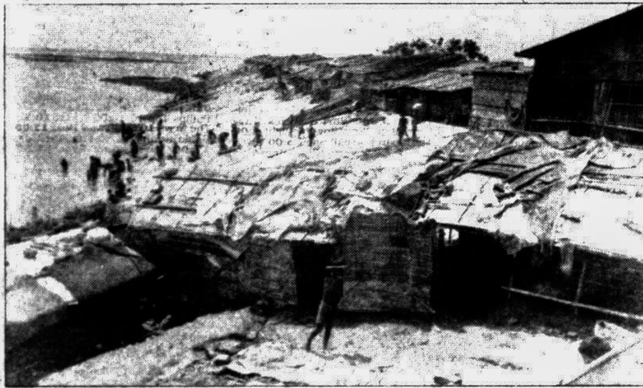
A large number of unauthorised shanties have recently cropped up on the Mohammadpur flood protection embankment. This photo was taken yesterday. — Star photo by Anisur Rahman
