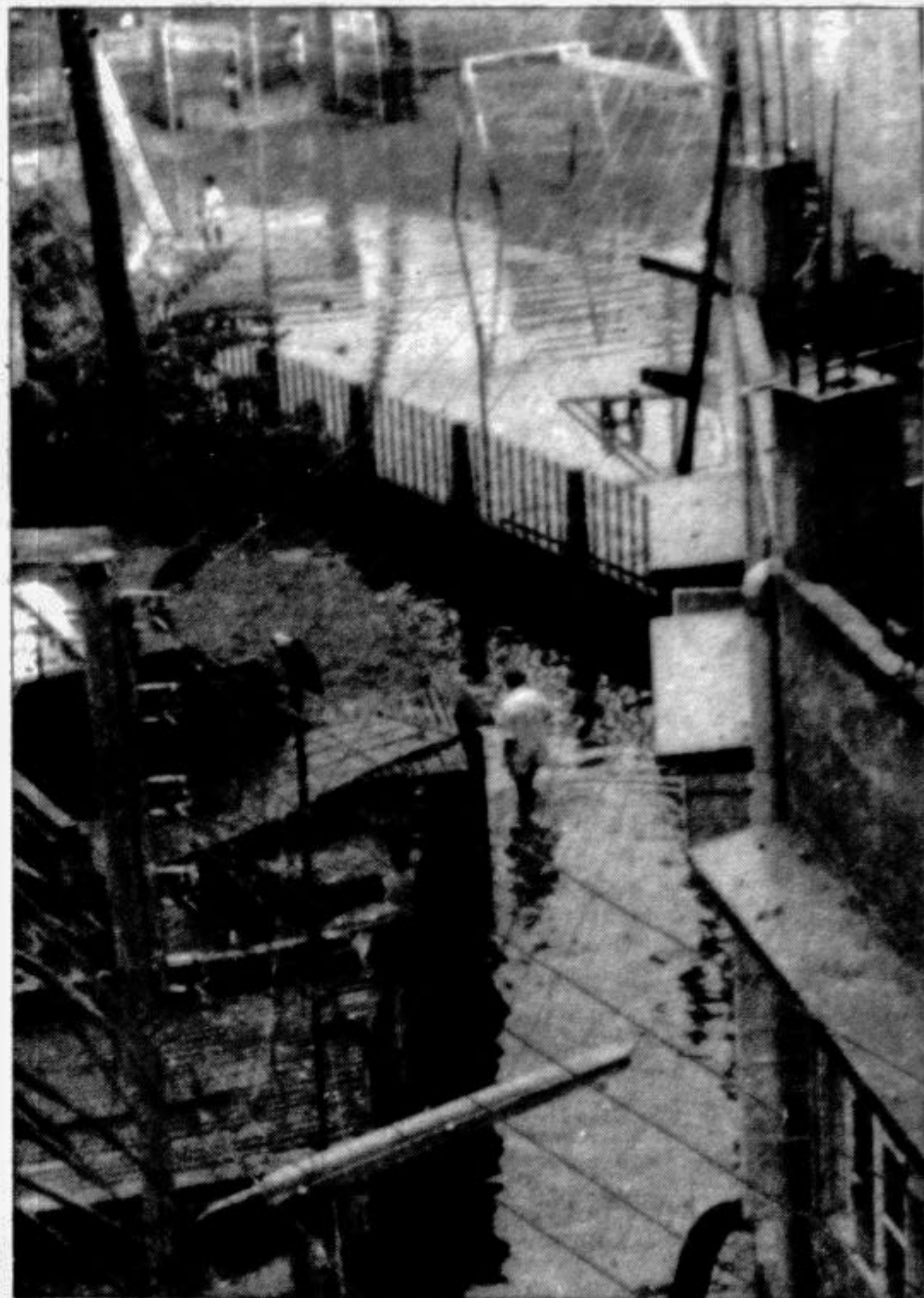
This picture, taken yesterday at Bahadurpur Lane of the city's Faridabad area, shows the extent of suffering caused to the residents due to water-logging even after a brief rainfall. - Star photo
