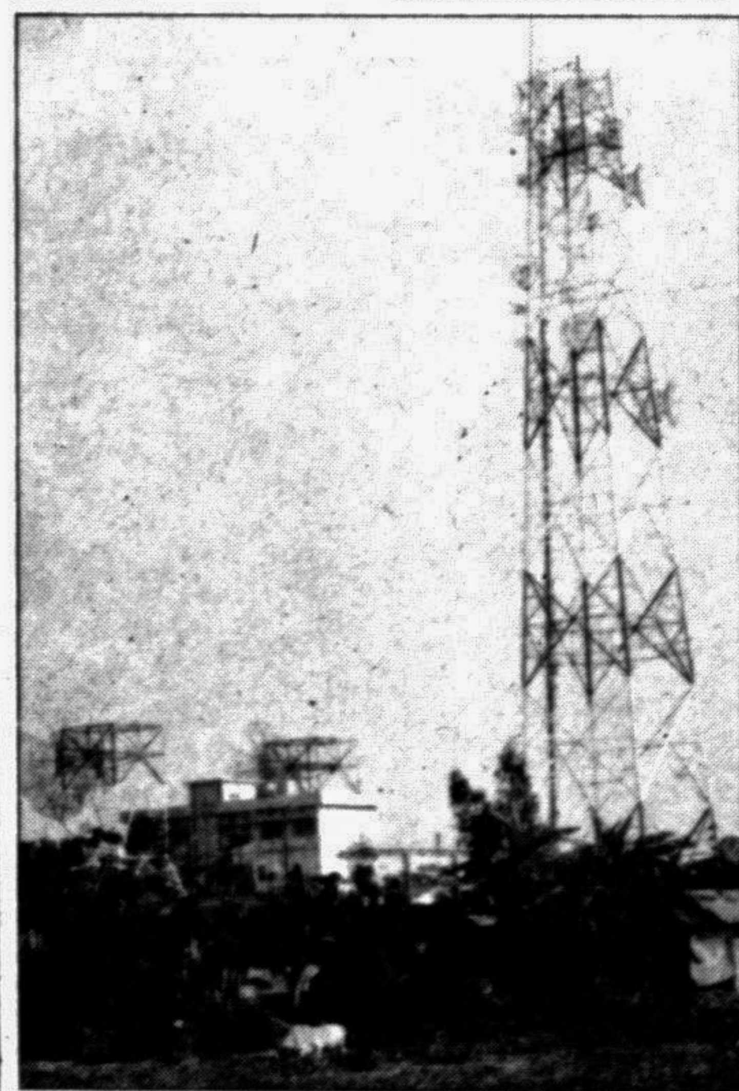
BARISAL: The T&T microwave tower at Barisal. — Star photo
