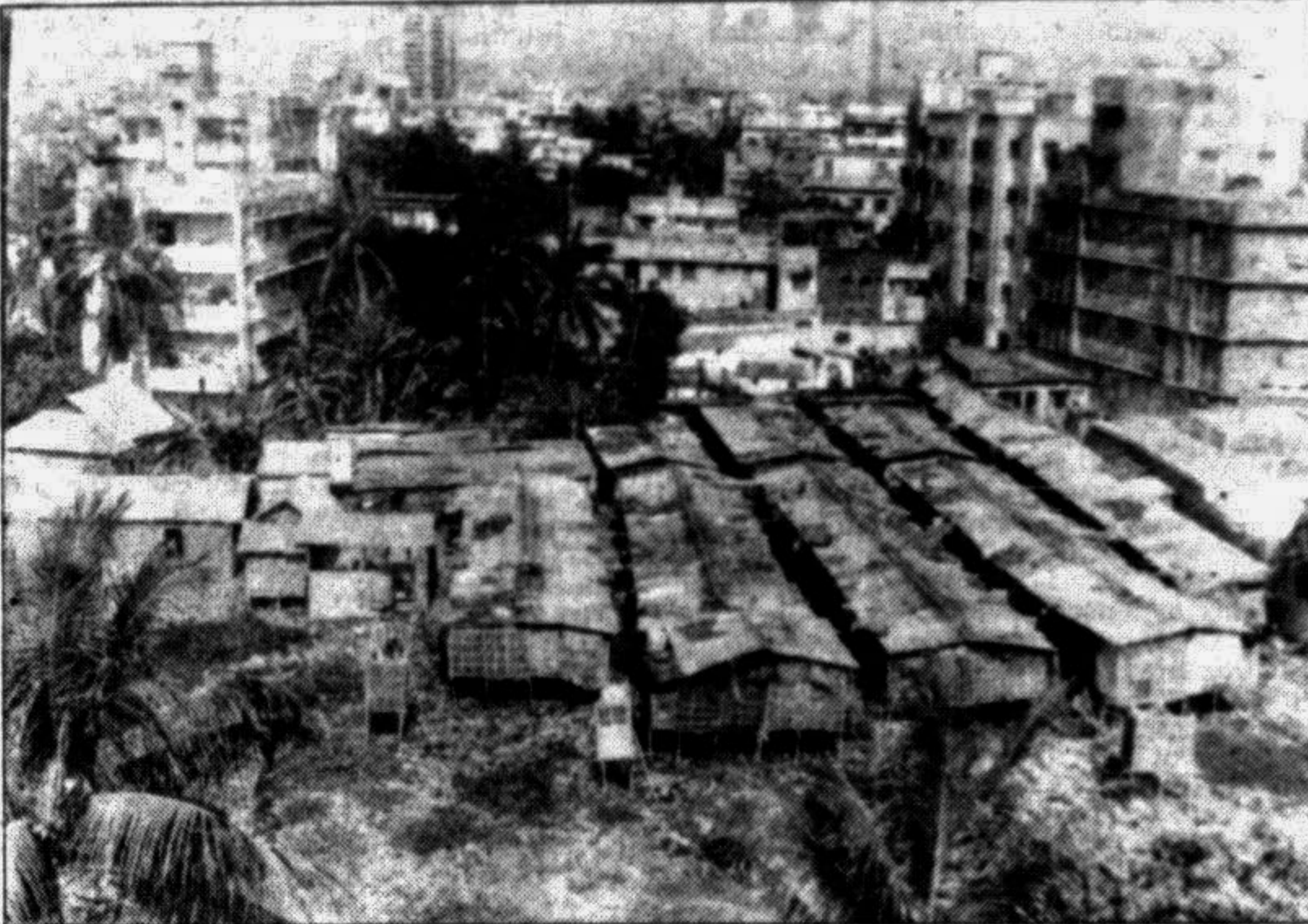
Such shanties on vacant plots in residential areas dotting the capital pose serious health and fire hazards and threats to law and order. — Staff photo
