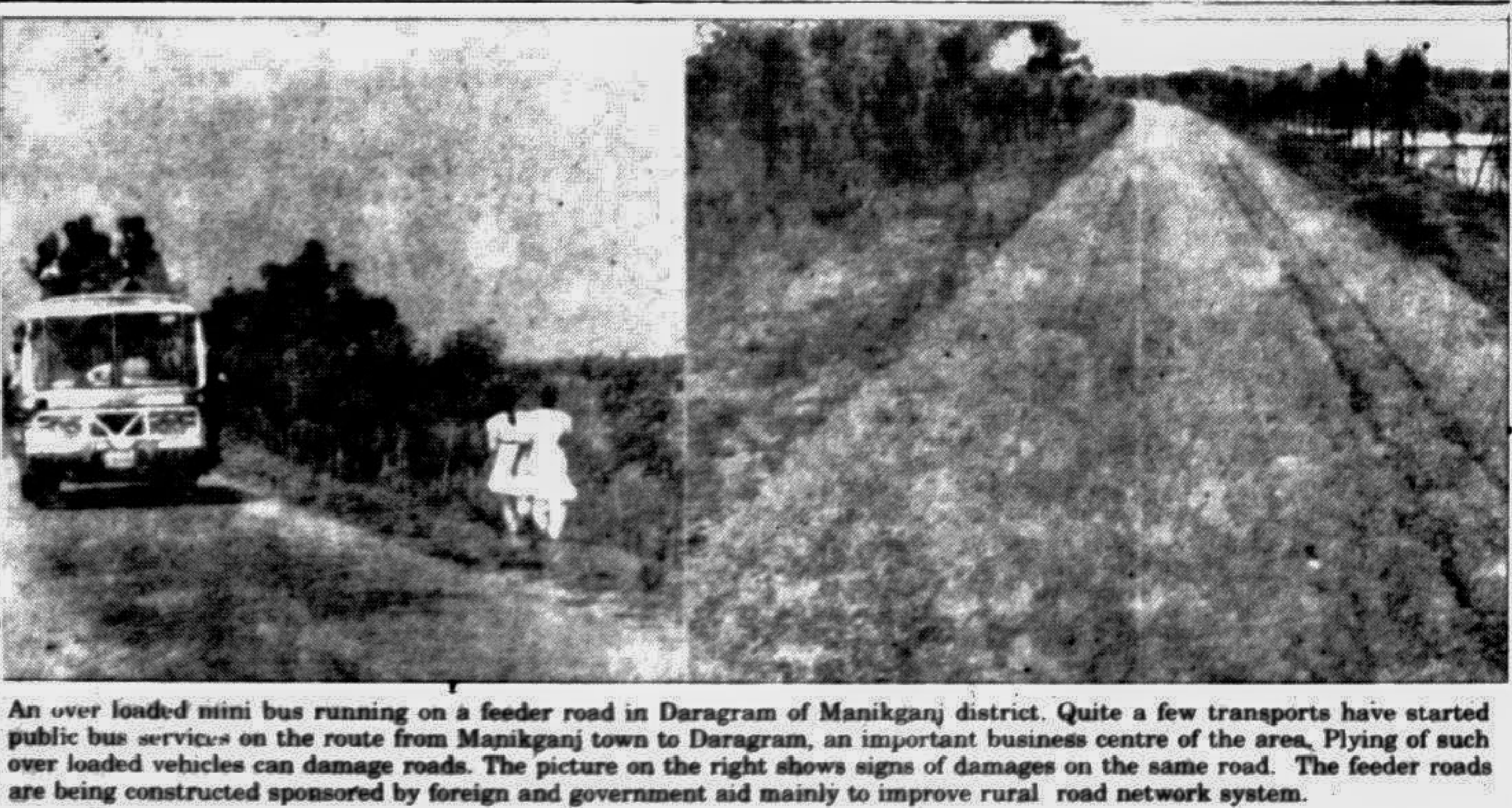
An over loaded mini bus running on a feeder road in Daragram of Manikganj district. Quite a few transports have started public bus services on the route from Manikganj town to Daragram, an important business centre of the area. Plying of such over loaded vehicles can damage roads. The picture on the right shows signs of damages on the same road. The feeder roads are being constructed sponsored by foreign and government aid mainly to improve rural road network system.
