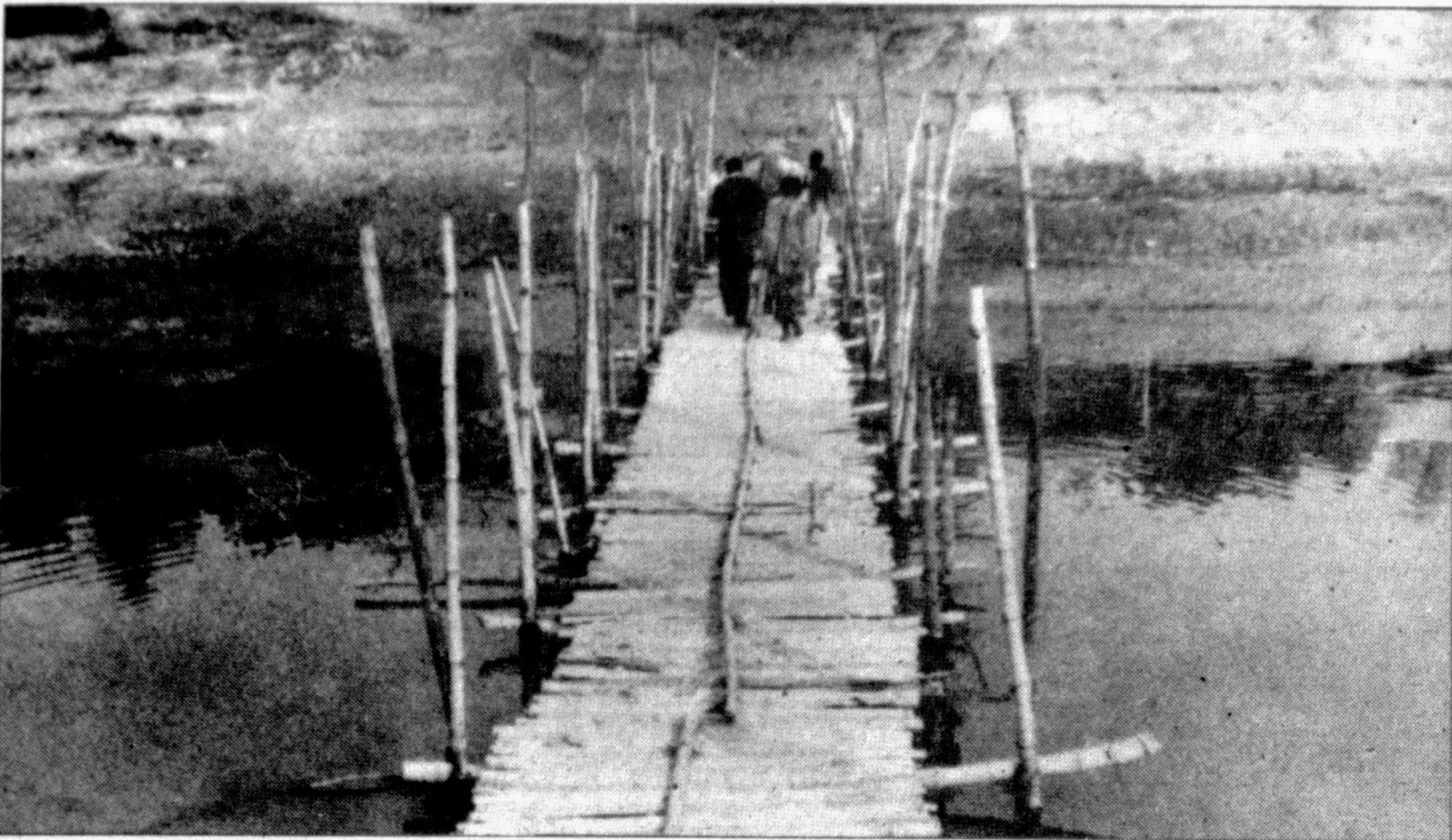
TANGAIL: A bamboo made bridge, in Nalnpara village, is mainly used for crossing of rickshaws and rickshaw vans. —Star photo
