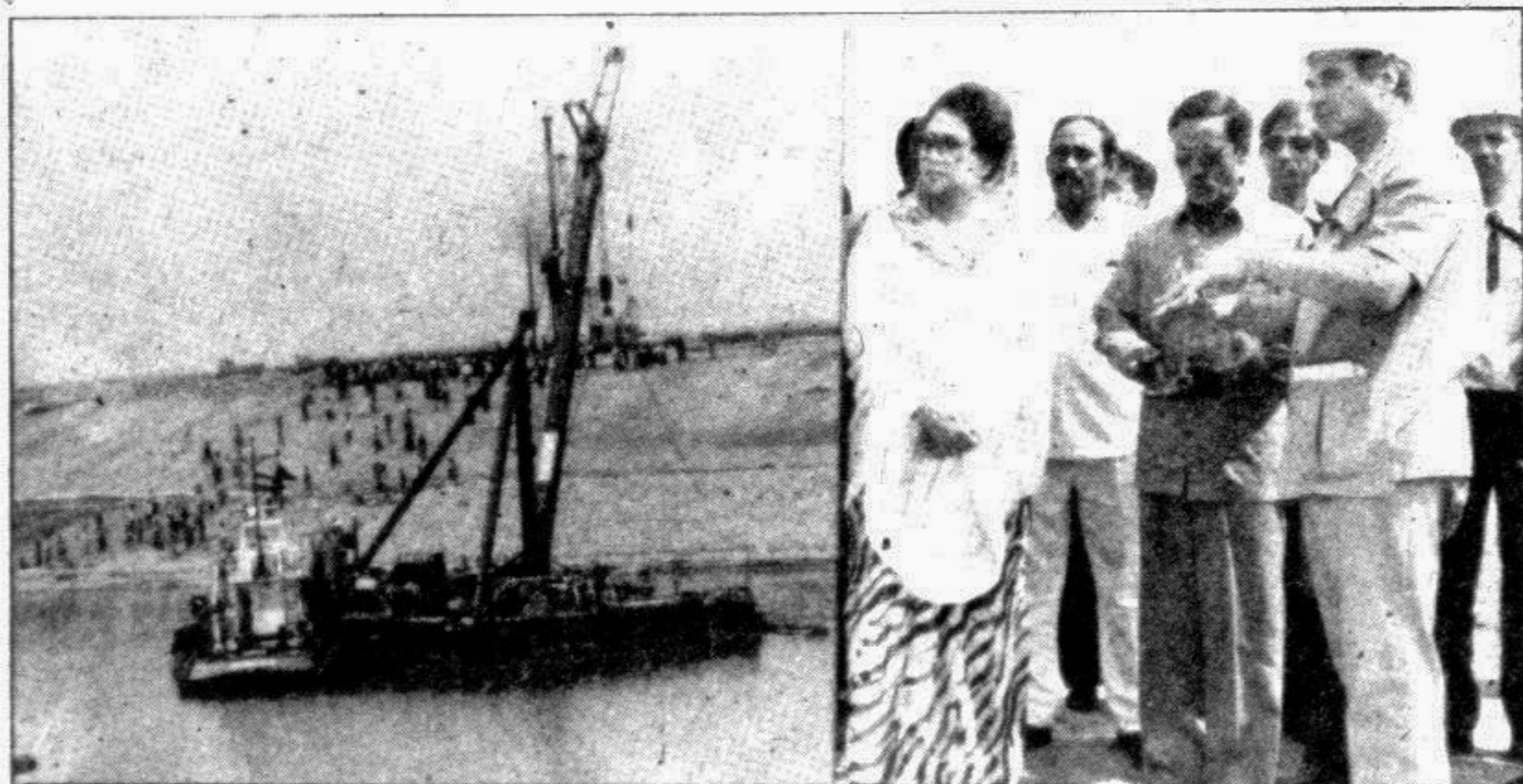
Prime Minister Begum Khaleda Zia being explained the dredging work at the construction site of the Jamuna multipurpose bridge at Kalihati in Tangail yesterday. She reviewed the progress of the physical construction of the JMB which began last October 16. — PID photo
