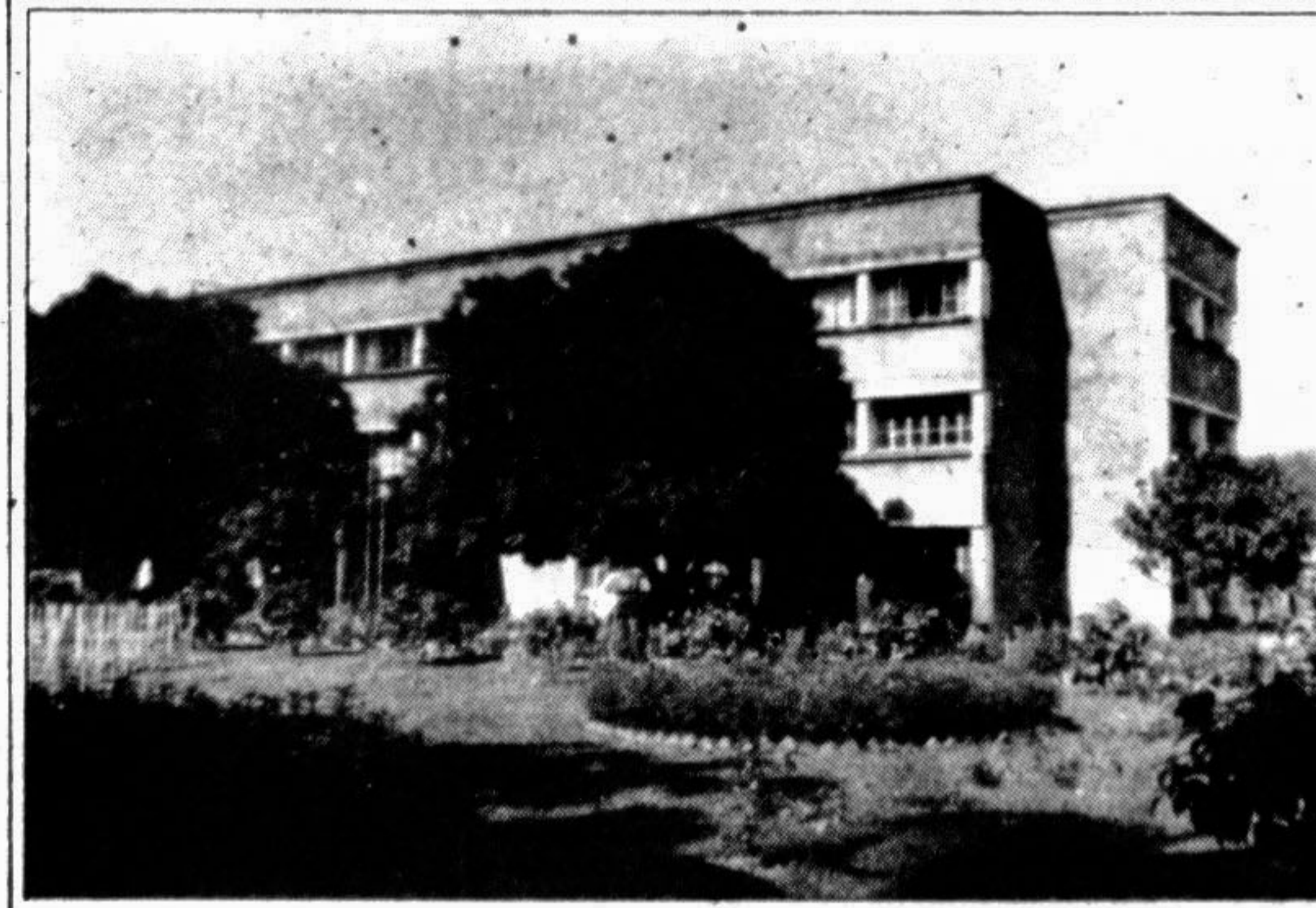
The Institute of Bangladesh Studies building inside the Rajshahi University campus. —Star photo
