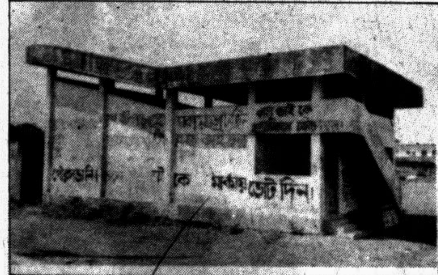
GOPALGANJ: The picture shows the squash game building constructed some ten years ago on ten kathas of land between the town stadium and the mosque in Bankpara. It is reported that the building was never used for the purpose it was built for. The building was constructed at the cost of Tk 3.75 lakh by the construction firm, Beta Syndicate. The officials of the firm claim that the concerned department has not yet paid the construction bill although construction of the building was completed. The building is now reportedly used for anti-social activities. —Star photo
