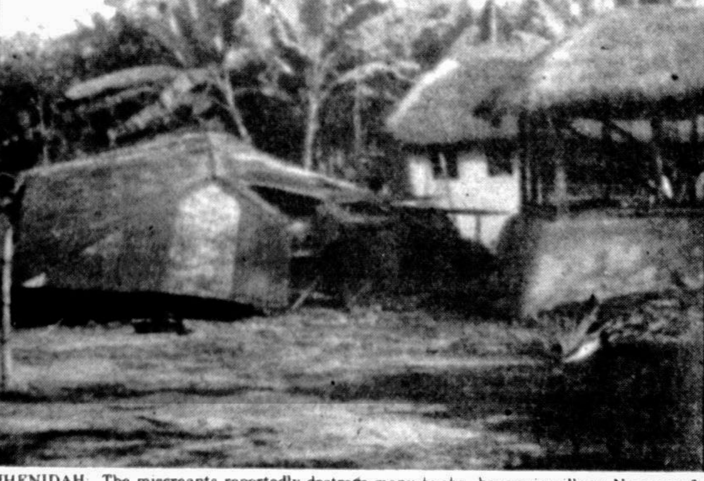
JHENIDAH: The miscreants reportedly destroys many kucha houses in village, Naopara of the district. The photo shows damaged house of Sher Ali Biswas. — Star photo
