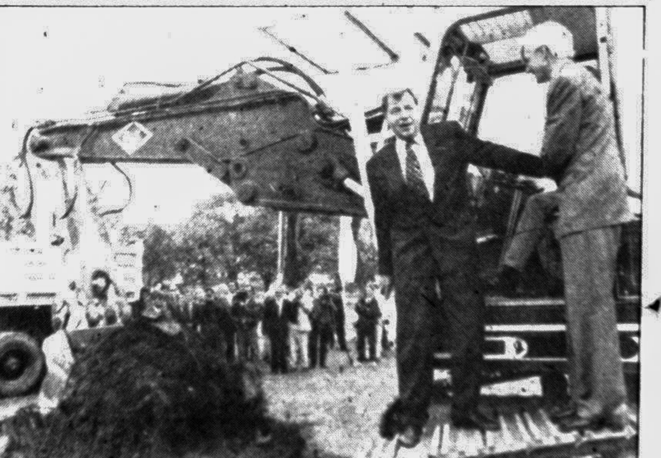
Big building site Berlin. On the Potsdamer Platz - in the centre of the city of millions - building work is going ahead at full speed, as Eberhard Diepgen, Berlin's Governing Mayor (Left), discovered. By 1998 about 7,500 people are to live and work here in an area of 340,000 square metres.
