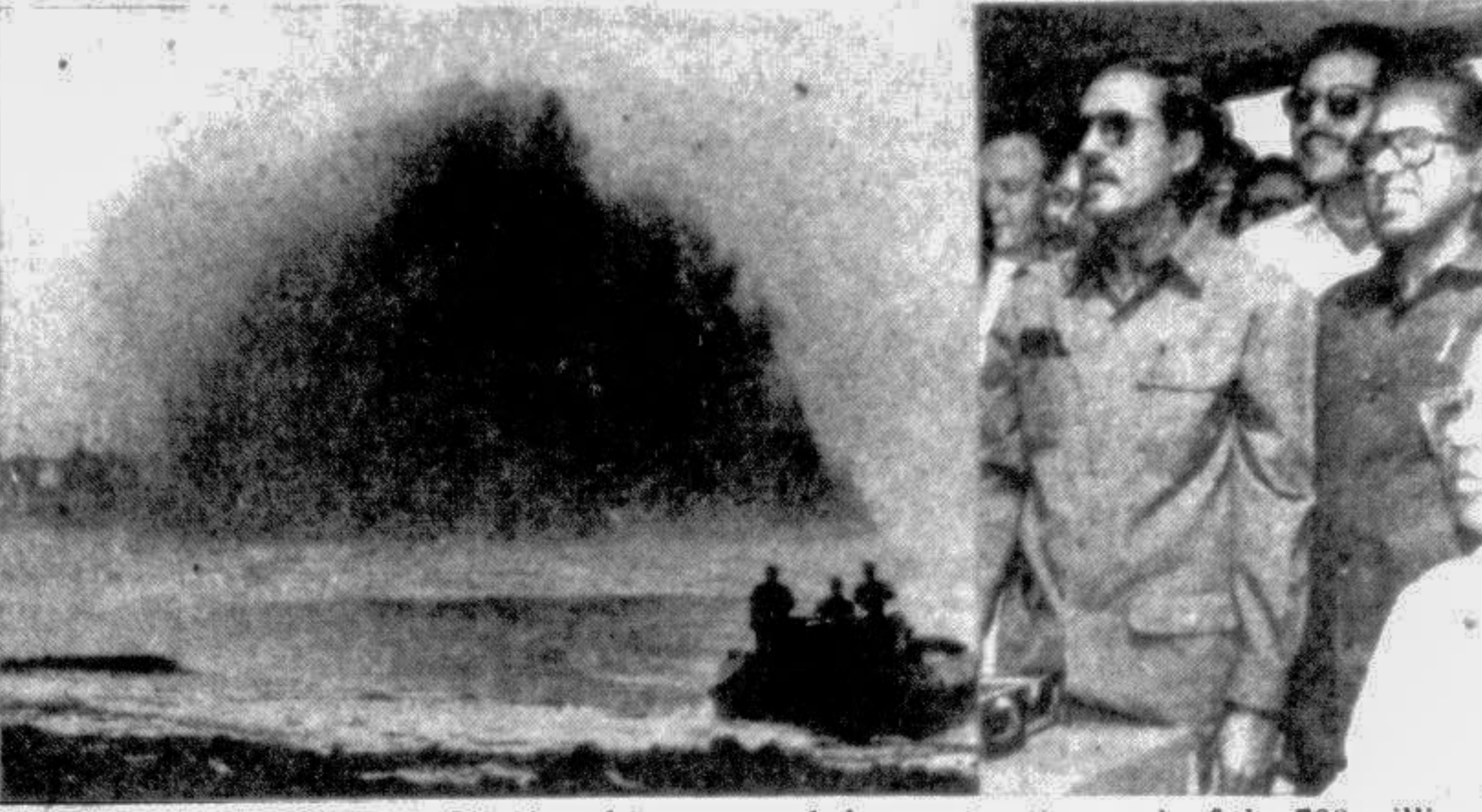
Communications Minister Oli Ahmed inaugurated the construction work of the 700-million US dollar Jamuna Multipurpose Bridge at Shyamshoil in Tangail yesterday by switching on a dredger (picture on left).
