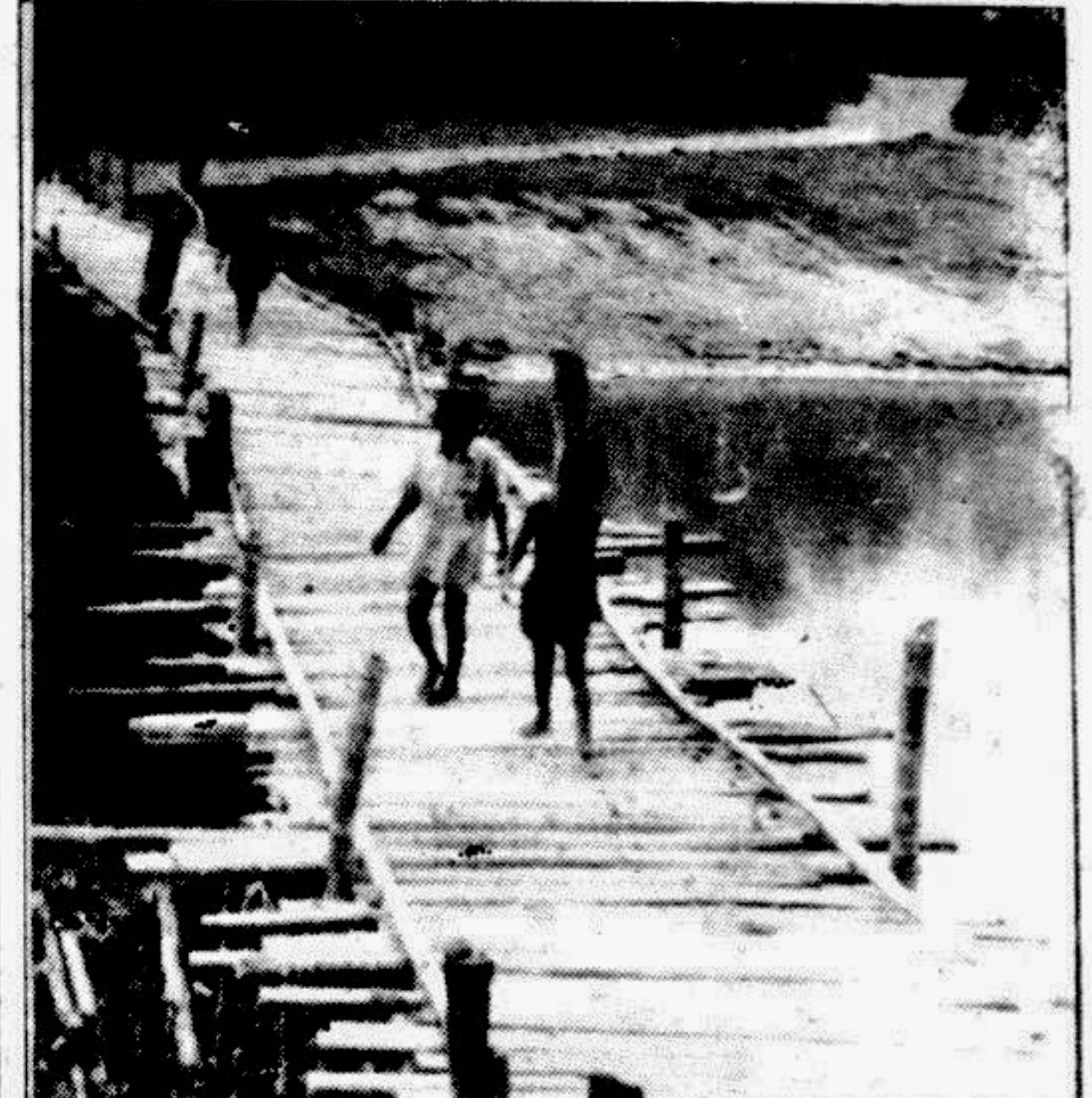
SHERPUR: A temporary bamboo bridge built at the initiative of the local people. This bridge connects a major business centre in the district town area. — Star photo
