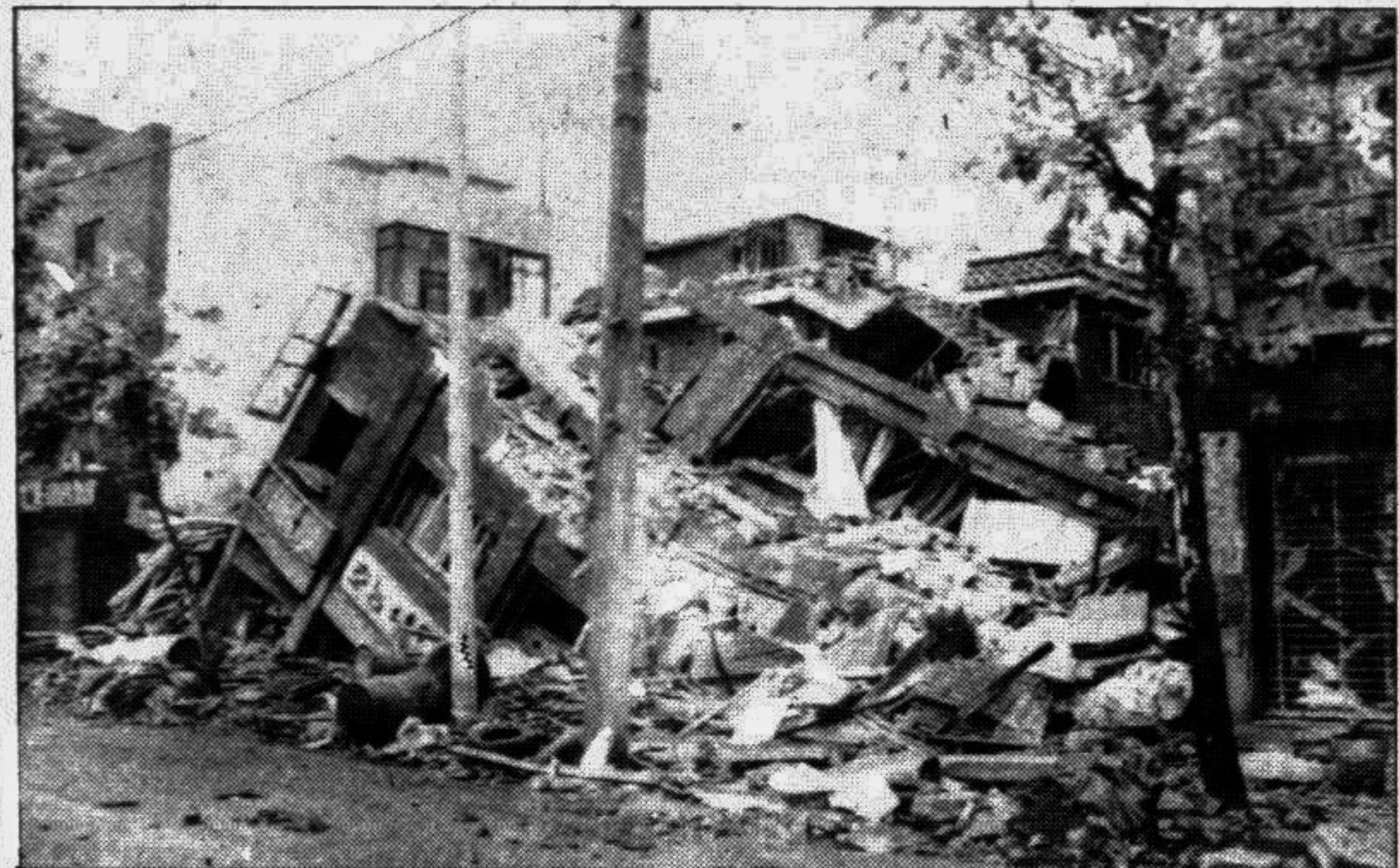
A four-story commercial building is a pile of rubble after an early morning cooking gas explosion toppled it, leaving six people seriously injured in the northern Tobong district in South Korea yesterday.
