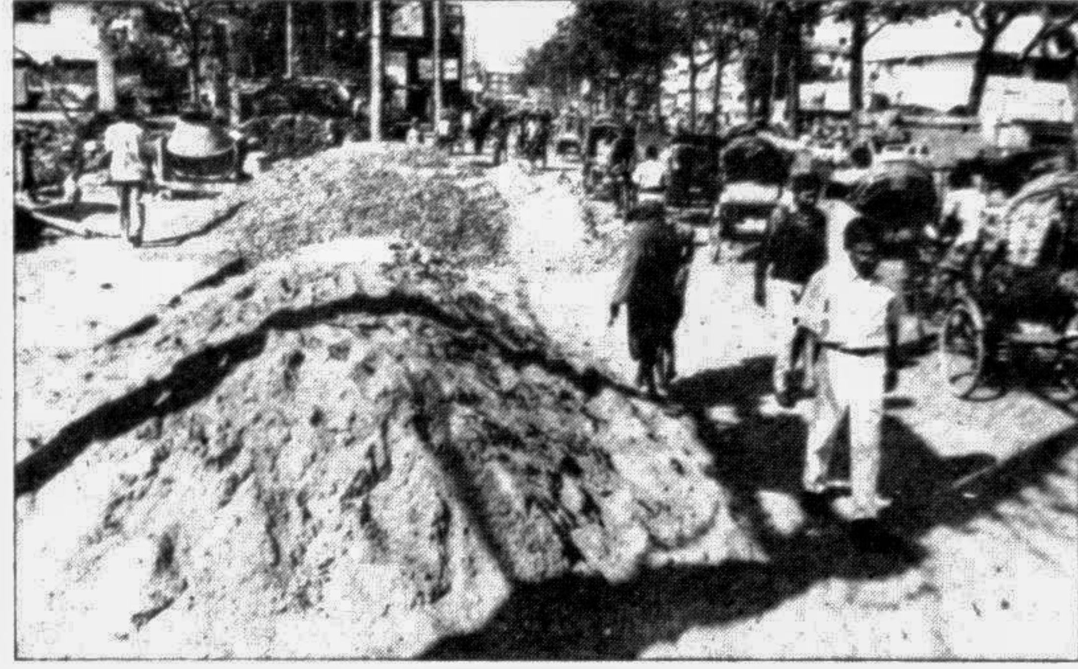
Construction material on the Bijoy Nagar Road near Puraña Paltan.
