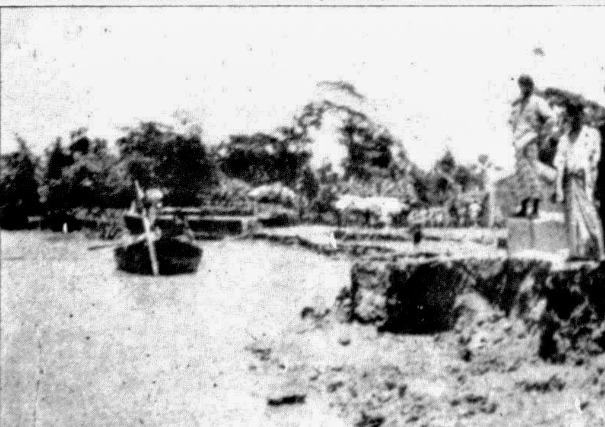
BARISAL: The river Kirtonkhola continues to engulf vast areas of land in the district. The photo shows a part of Charkaua area hit by the river erosion. — Star photo
