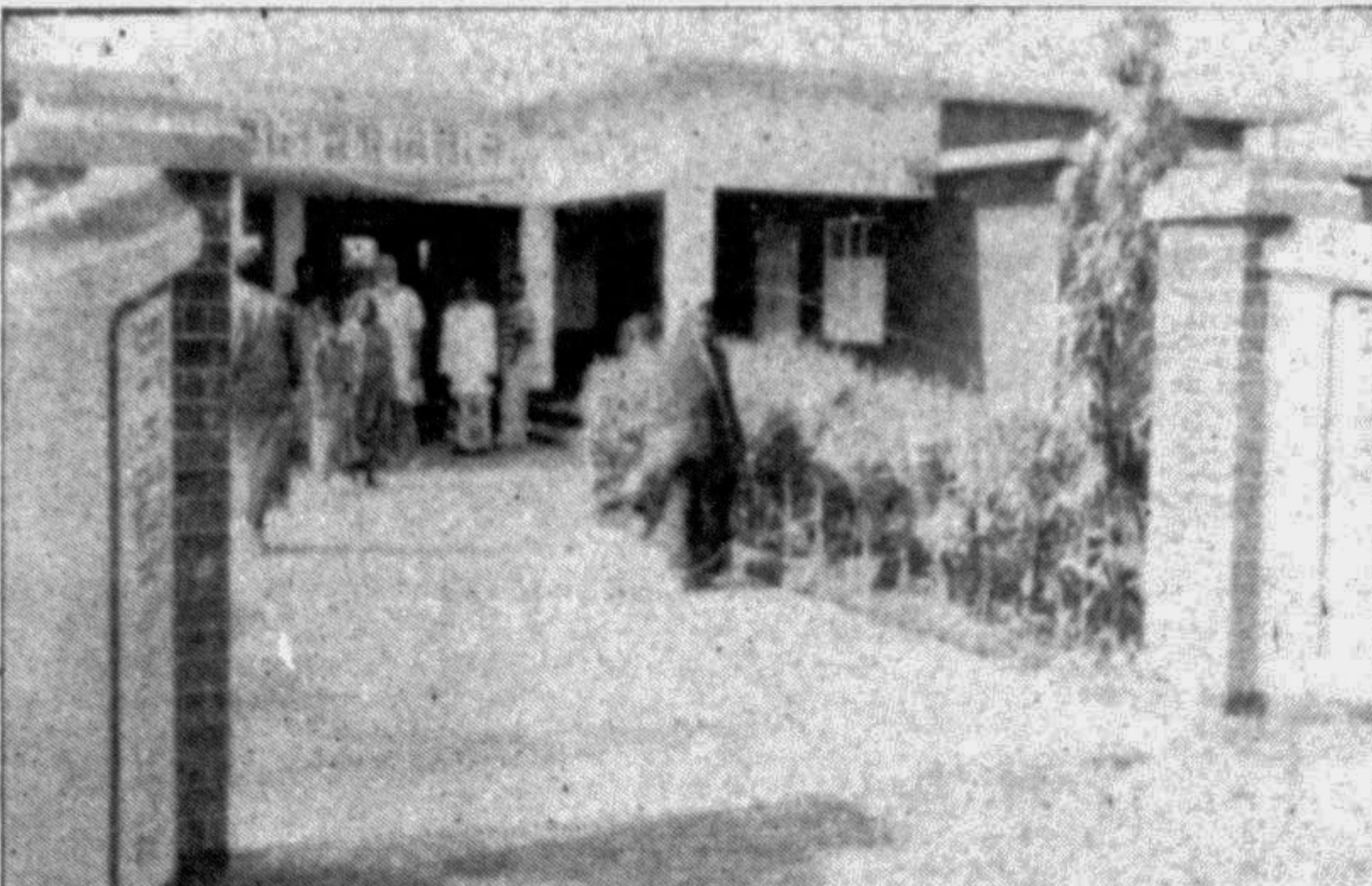
RANGPUR: The newly constructed hospital-cum-clinic, Hena Memorial Hospital at Rangapur in Mithapukur thana so far offered treatment to some 22,000 patients free of cost. The 33-bed hospital cost Taka 30 lakh to construct which was provided by a local industrialist and social worker. — Star photo
