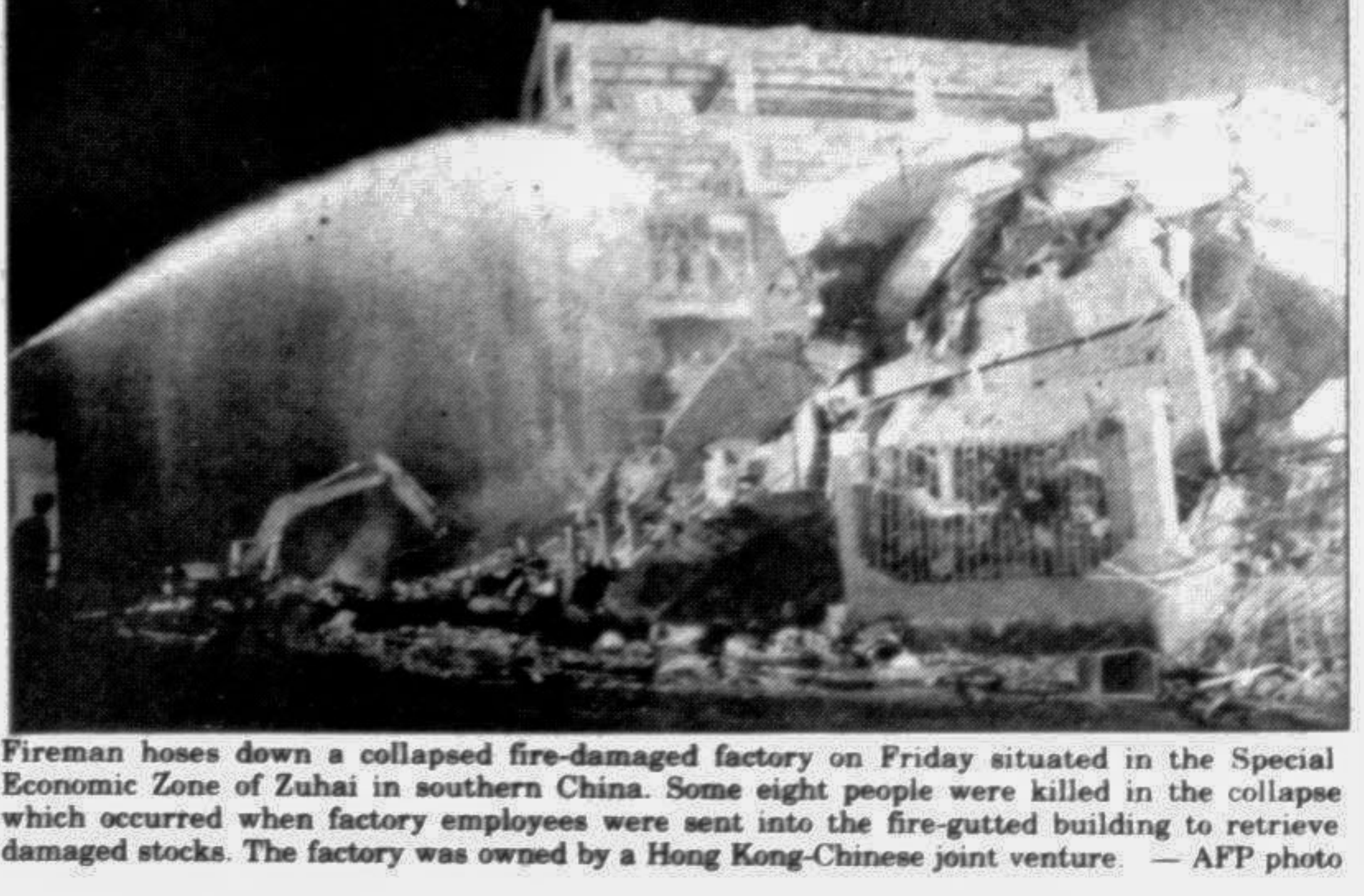
Fireman hoses down a collapsed fire-damaged factory on Friday situated in the Special Economic Zone of Zuhai in southern China. Some eight people were killed in the collapse which occurred when factory employees were sent into the fire-gutted building to retrieve damaged stocks. The factory was owned by a Hong Kong-Chinese joint venture. — AFP photo
