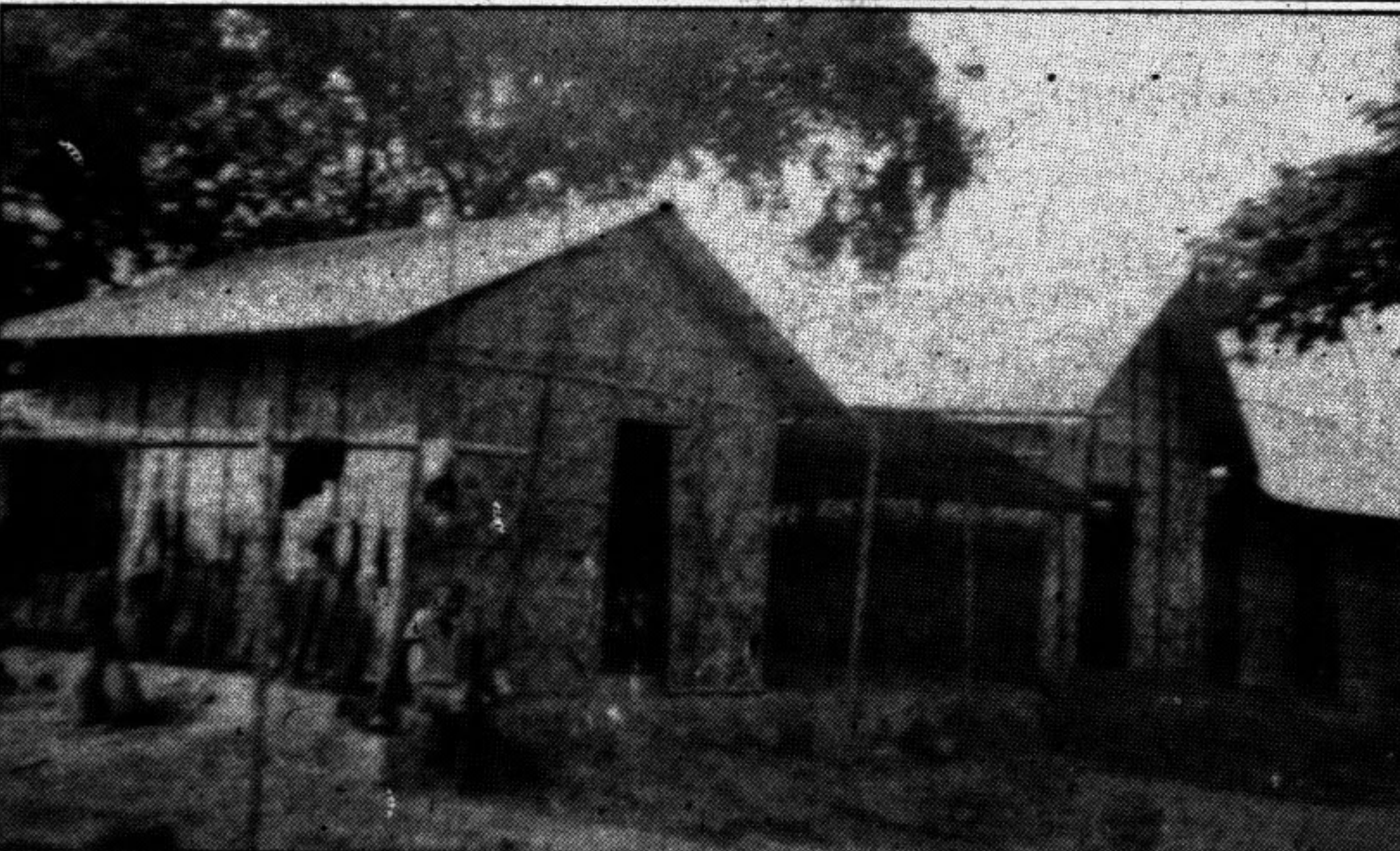
SYLHET: An international Islamic organisation has constructed 39 kuncha houses in Balaganj village of the district recently, under its flood rehabilitation programme. — Star photo
