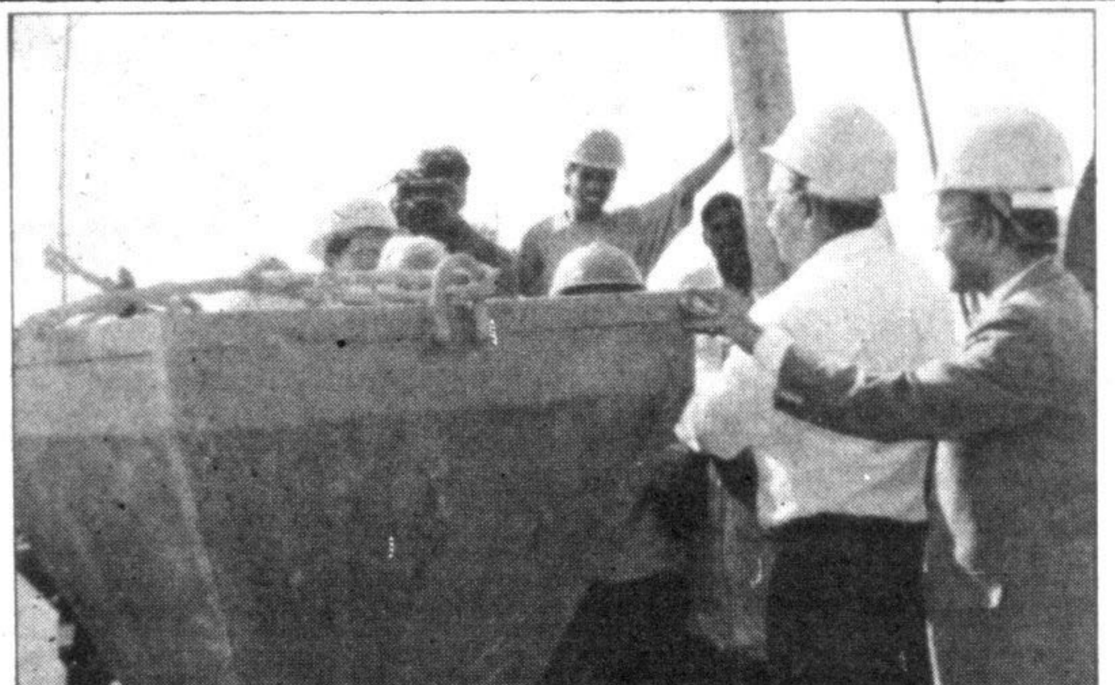
Finance Minister M Saifur Rahman inaugurating the piling work of Sylhet 90 MW Combined Cycle Power Plant Project at Fenchuganj on Nov 25. Energy and Mineral Resources Minister Dr Khondaker Mosharraf Hossain is seen in the picture.
