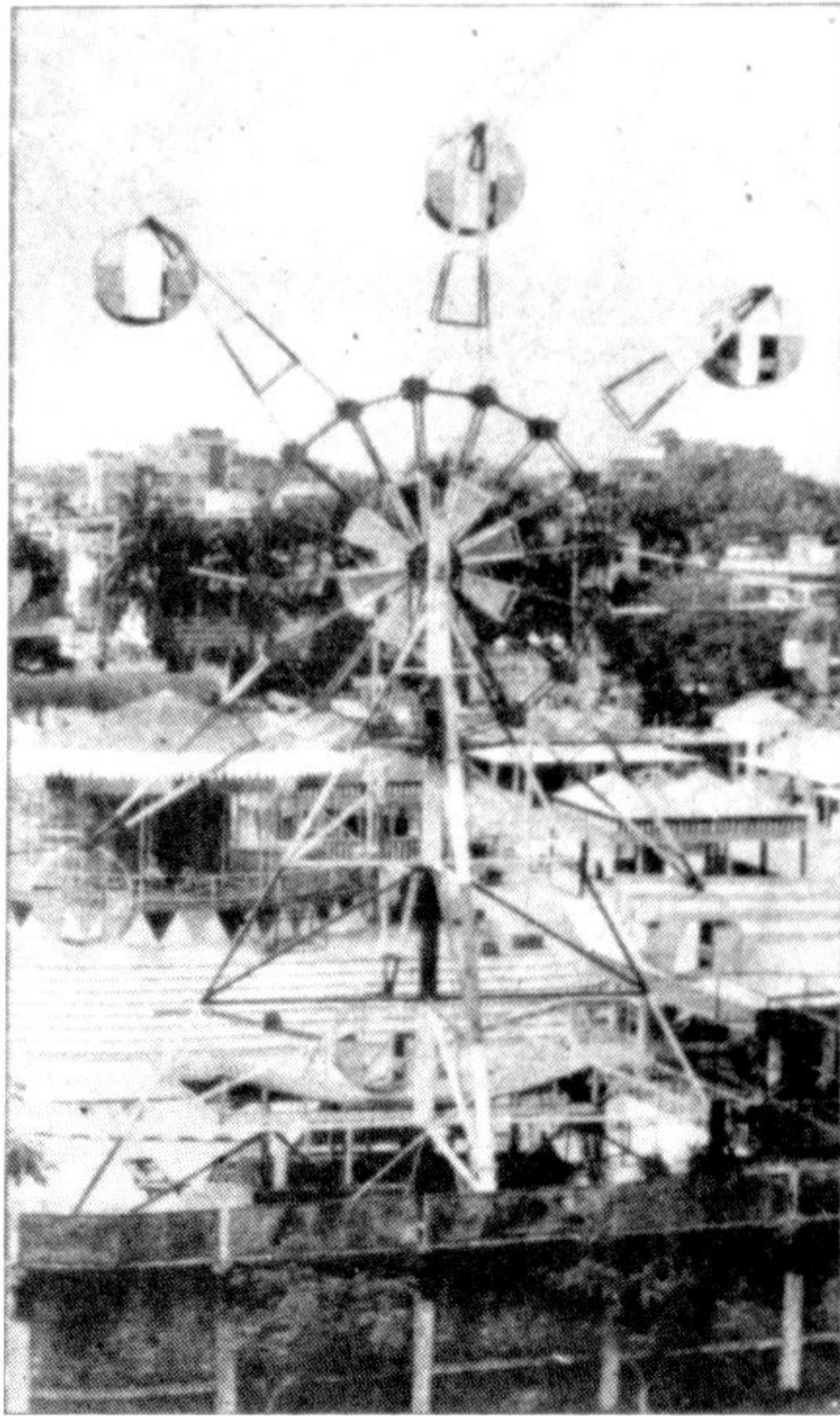
View of an under-construction private sector children's and amusement park near the Orthopaedics (Pangu) Hospital at Shyamoli in the city. — Star photo
