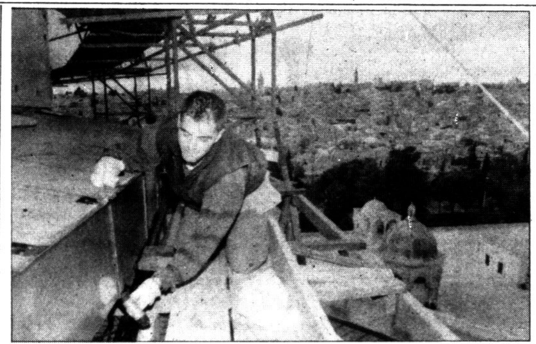
An Irish worker fixes a gold-layered plate onto the Dome of the Rock mosque in Jerusalem Thursday on the Mosques compound, the third holiest site in Islam. As part of a multi-million dollar restoration project, the Mivan company from northern Ireland is putting a fine layer of 24-carat gold on the seventh century shrine from which Muslims believe Mohammad made his night journey to heaven.
