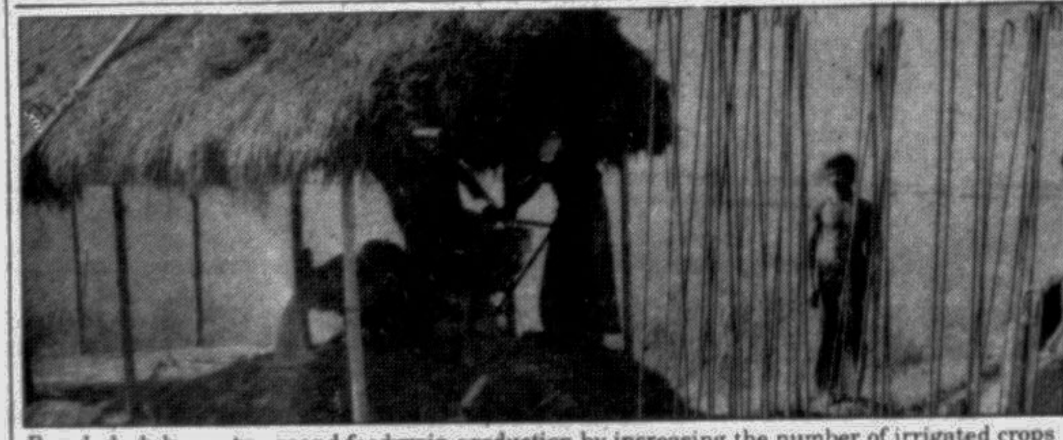
Bangladesh hopes to expand foodgrain production by increasing the number of irrigated crops and using its irrigation facilities more effectively. A sturdy junction box of reinforced concrete is being built to direct the water which will soon flow from the pump under the roof in the background.
