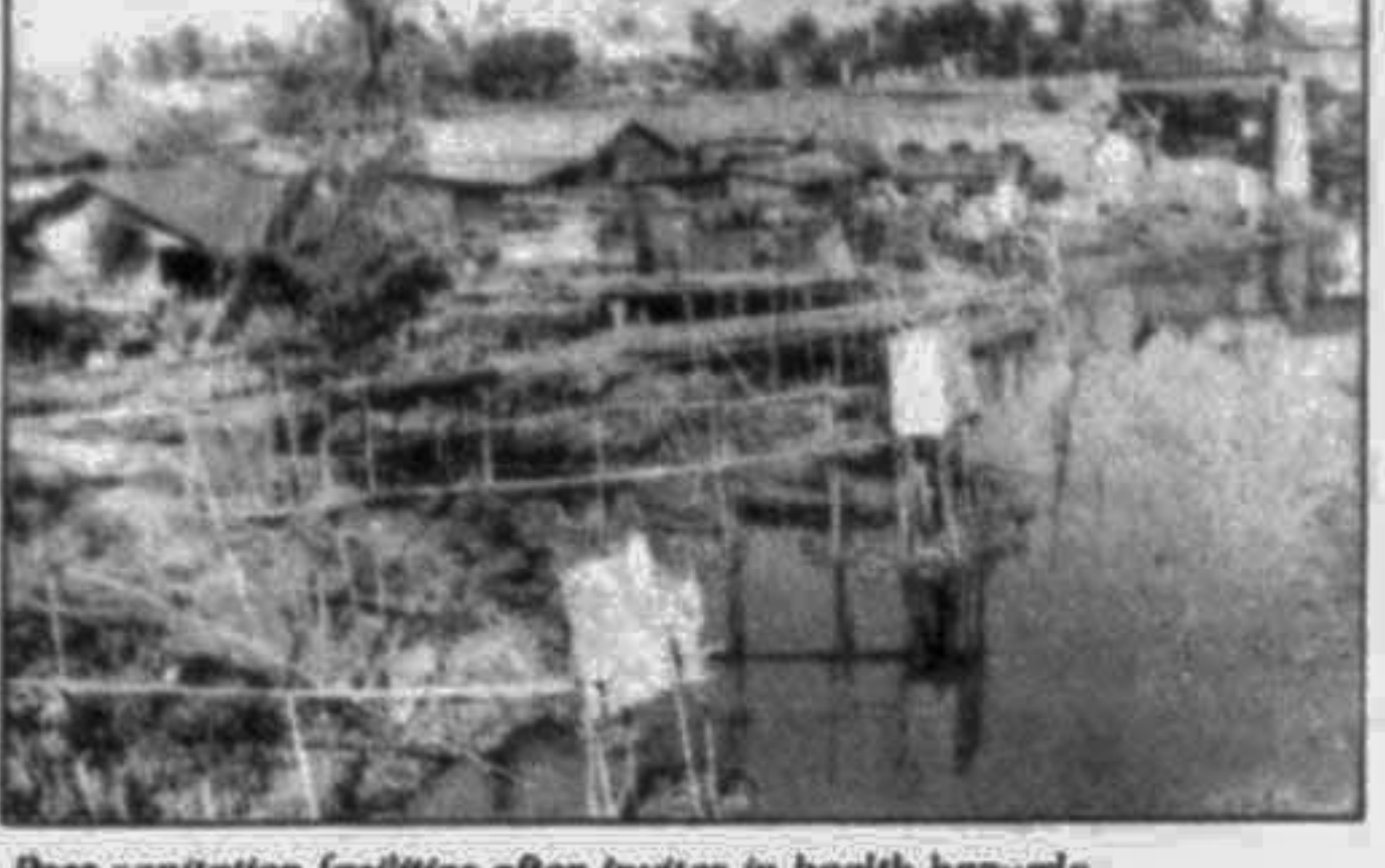
Poor sanitation facilities often invites in health hazards. — Star photo
