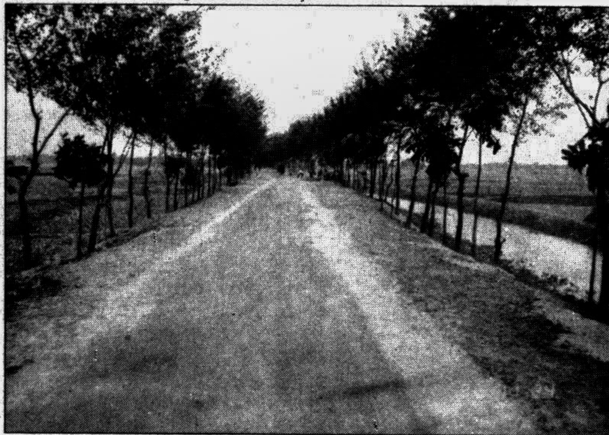
Rural road connecting Homna growth centre to Dhaka-Chittagong Highway.
