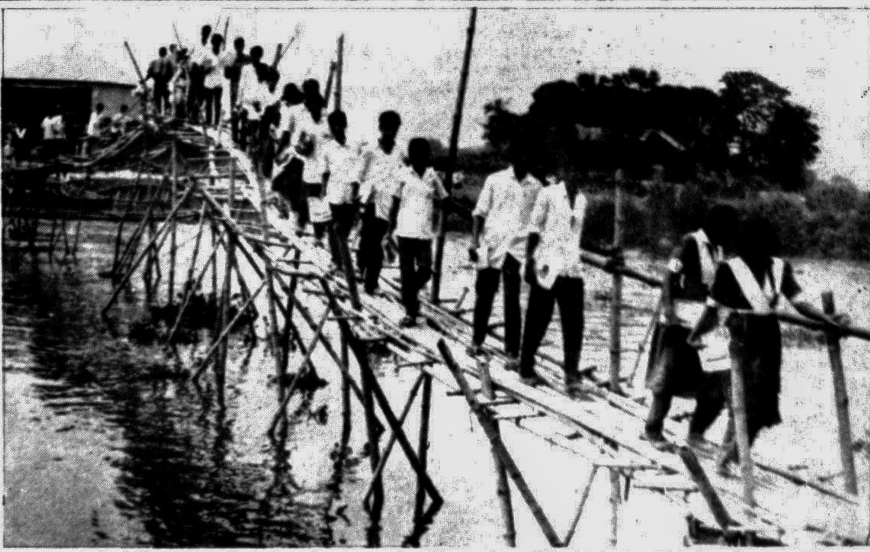
These school children cross this bridge almost everyday. The condition of the bridge is said to be quite poor. A large number of people also use the bridge located in Demra Thana.
