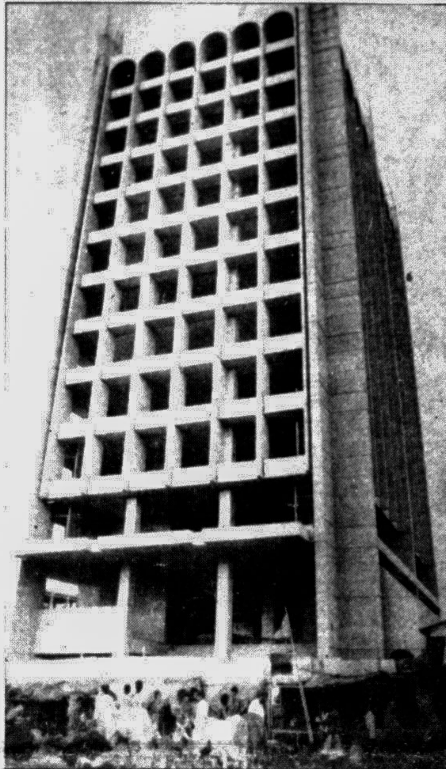
The Janata Tower at Kawran Bazar — Star photo
