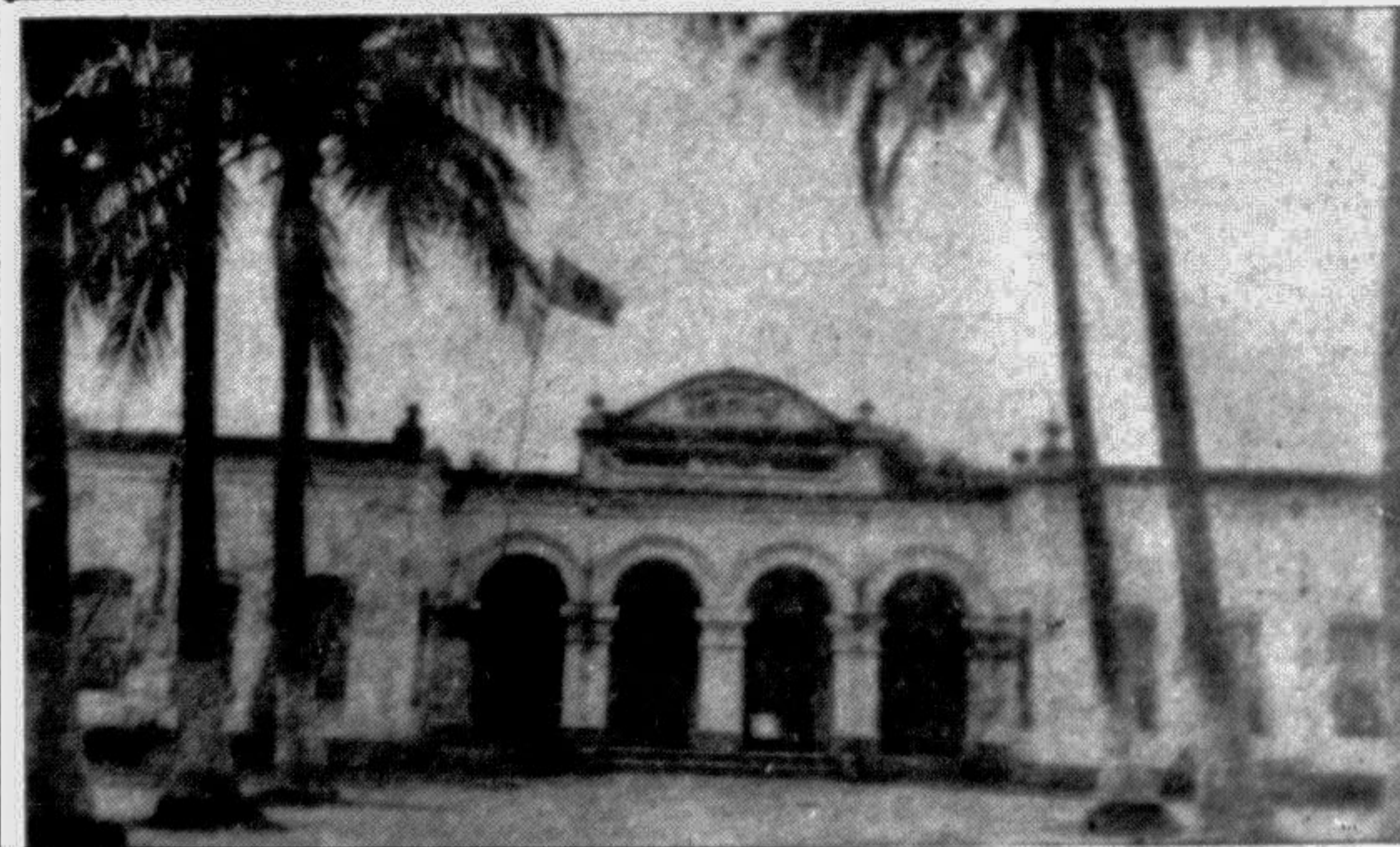
PABNA: Pabna Gopal Chandra Institution, a century-old secondary high school requires immediate renovation. — Star photo
