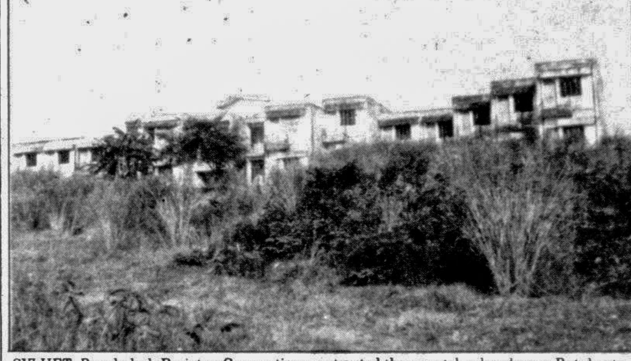
SYLHET: Bangladesh Parjatan Corporation constructed these motel a decade ago. But due to unknown reasons, it is still lying unused. — Star photo
