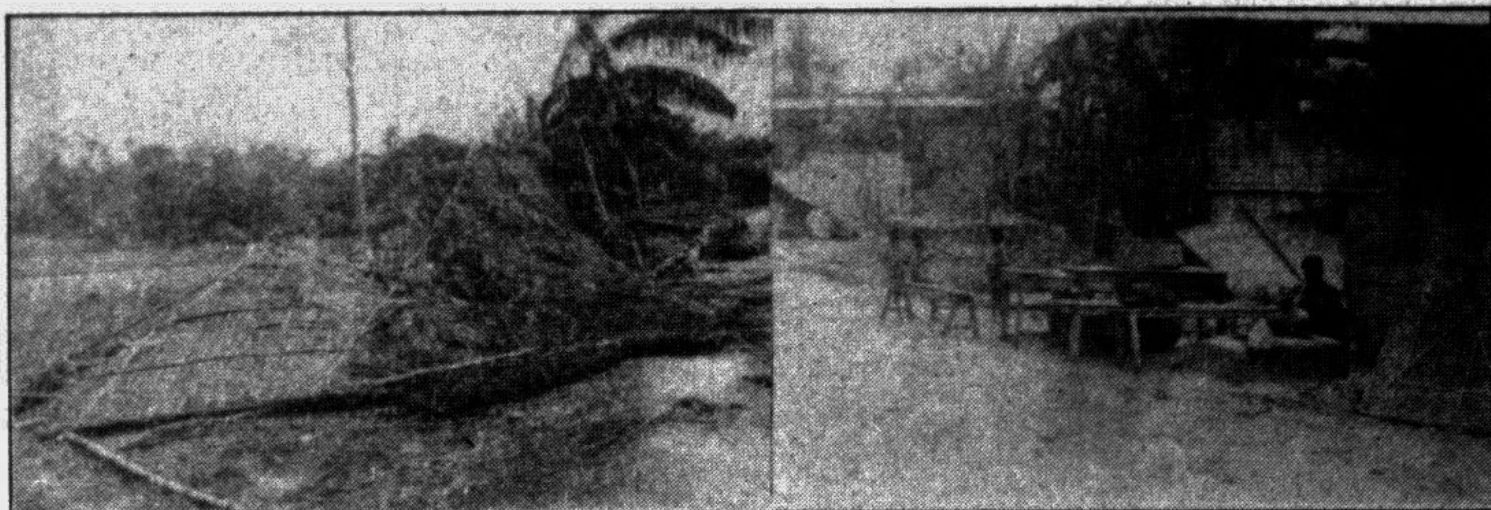
JAMALPUR: The cyclonic storm that hit Mahdan union under Sarishabari thana of the district damaged most of the kancha houses on January 8. —Star photo
