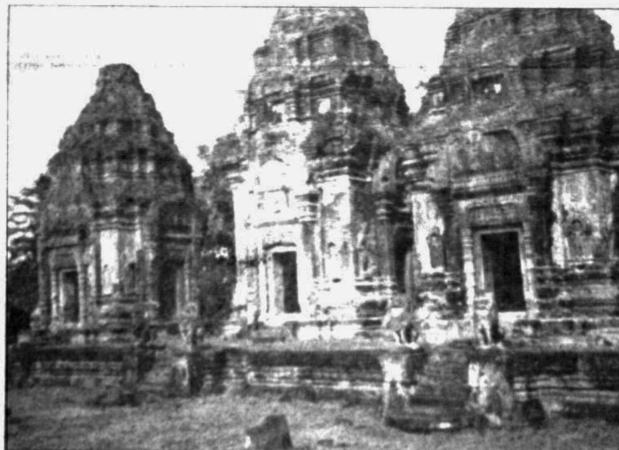
The ninth century temples were finished in brick with laterite cores. As the skills of the woodcarvers were taken up by the stonemasons, the use of sandstone became general, the stone being brought some distance by elephant.
