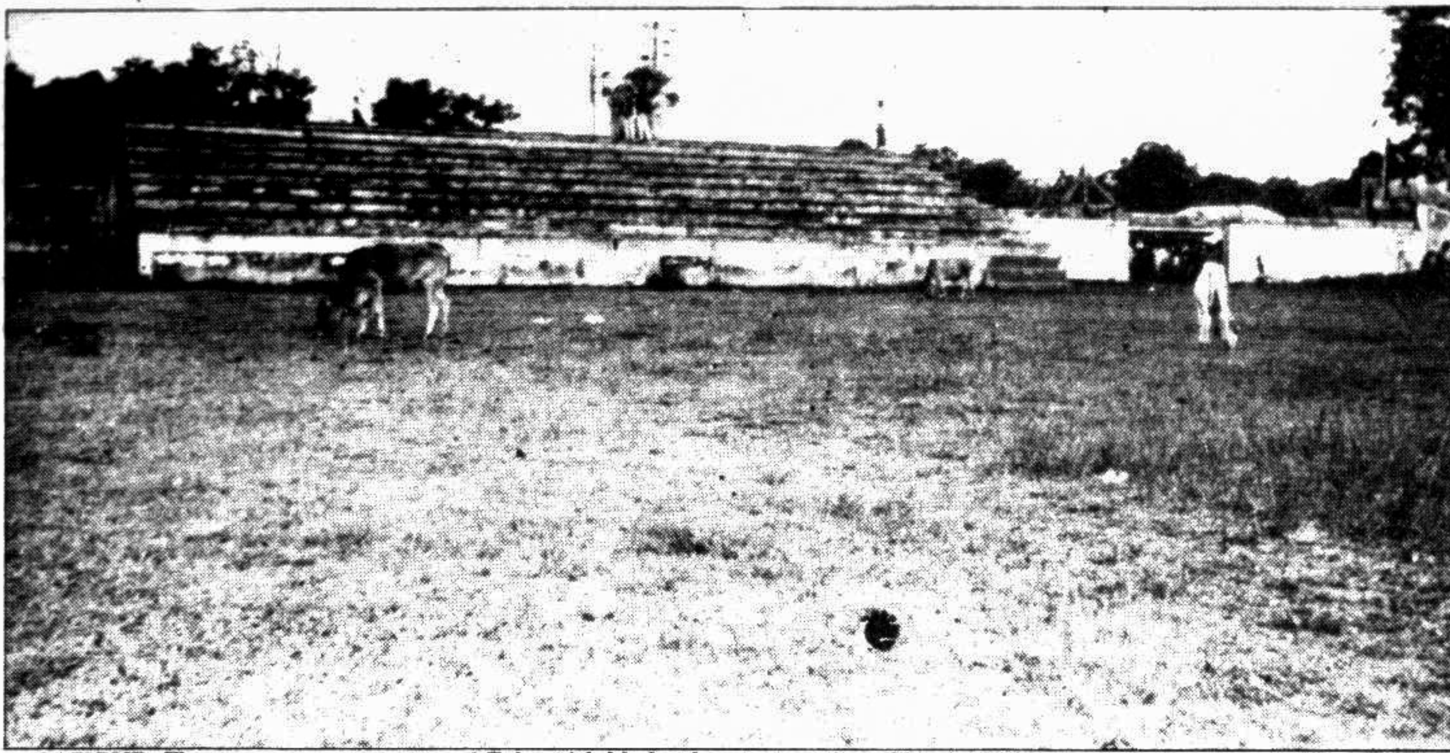
GAZIPUR: The government sanctioned Taka 10 lakh for the construction of local stadium in 1982. But the work is yet to be completed after expiry of 12 years. — Star Photo
