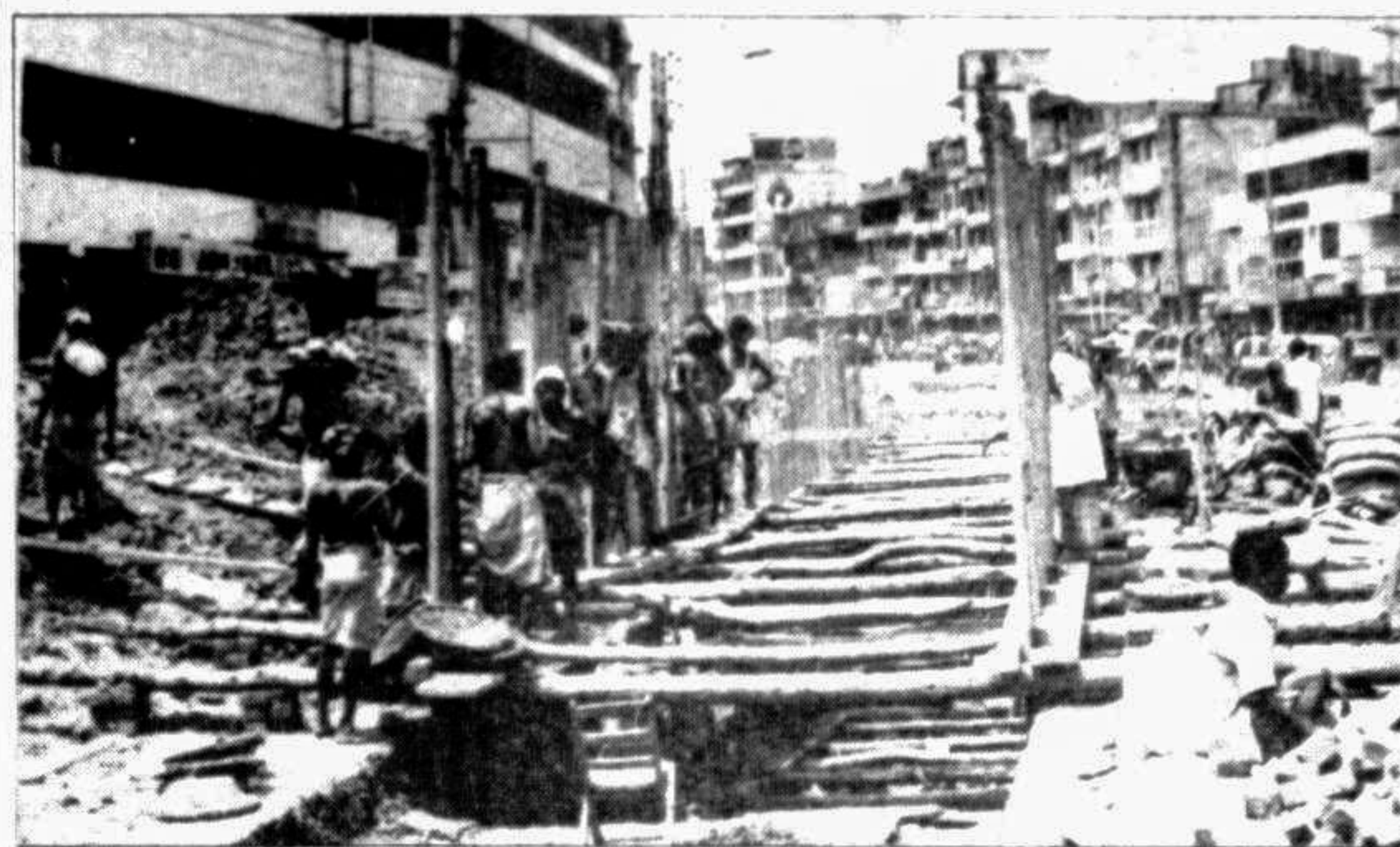
Construction of storm sewer in progress.
