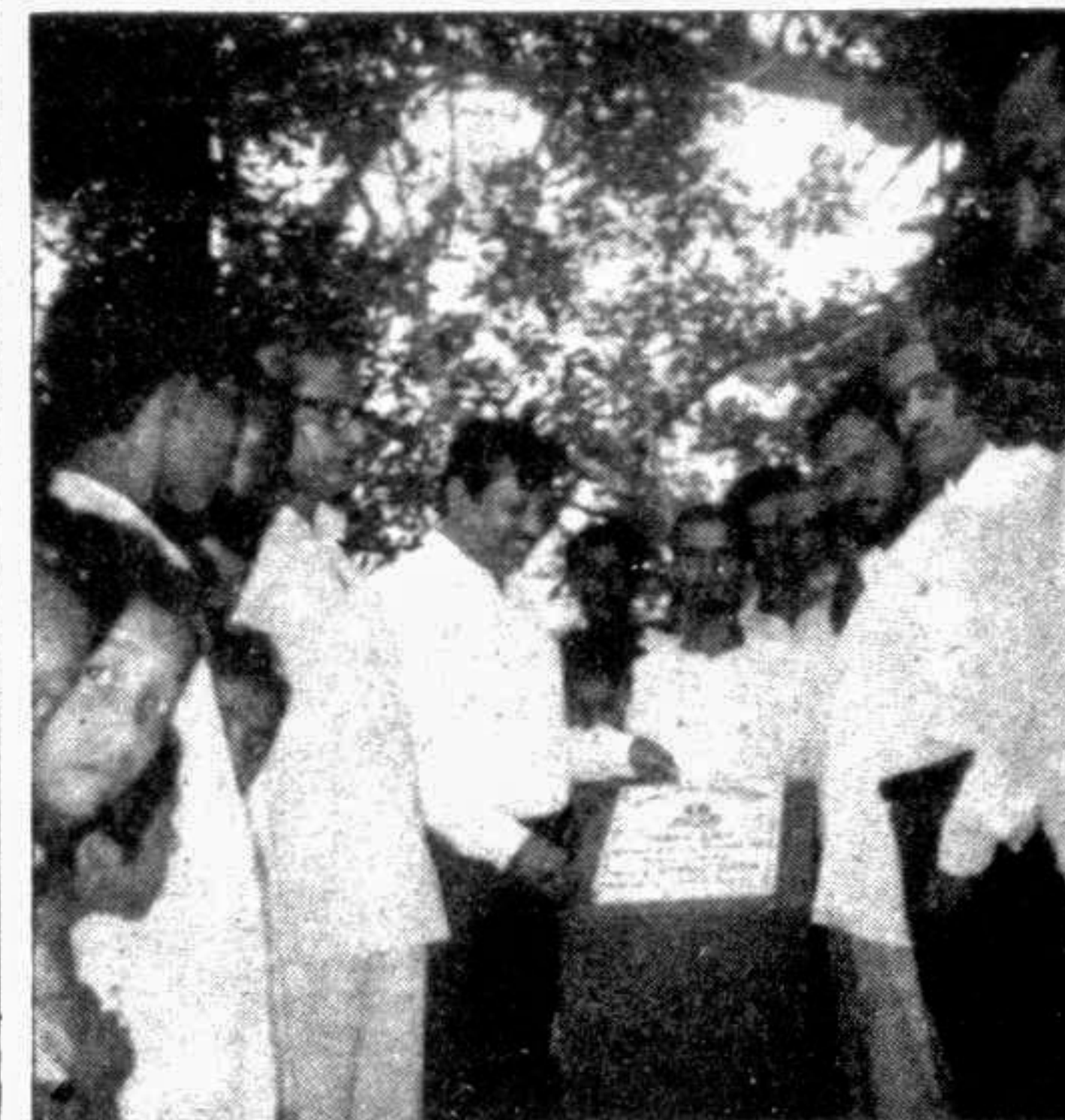
Ln. Humayun Zahir, District Governor District-315A, laying the foundation stone of LCIF funded Science Building cum Cyclone shelter of Sonapur High School at Begumganj, Noakhali on Sunday.
