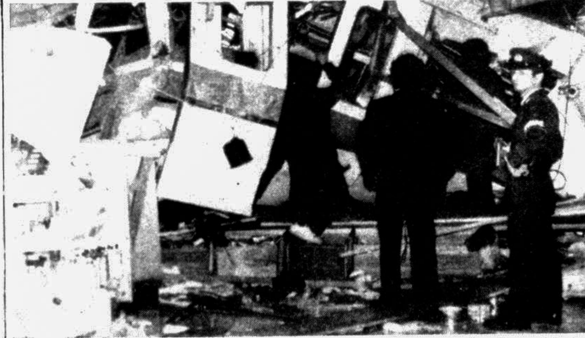
TORIDE, JAPAN: Local authorities investigate the wreckage of a train that slammed into a store in the terminal station building Tuesday after overrunning the tracks, in Toride, Ibaraki prefecture. One passenger was killed and 158 other commuters were injured in the early morning accident.
