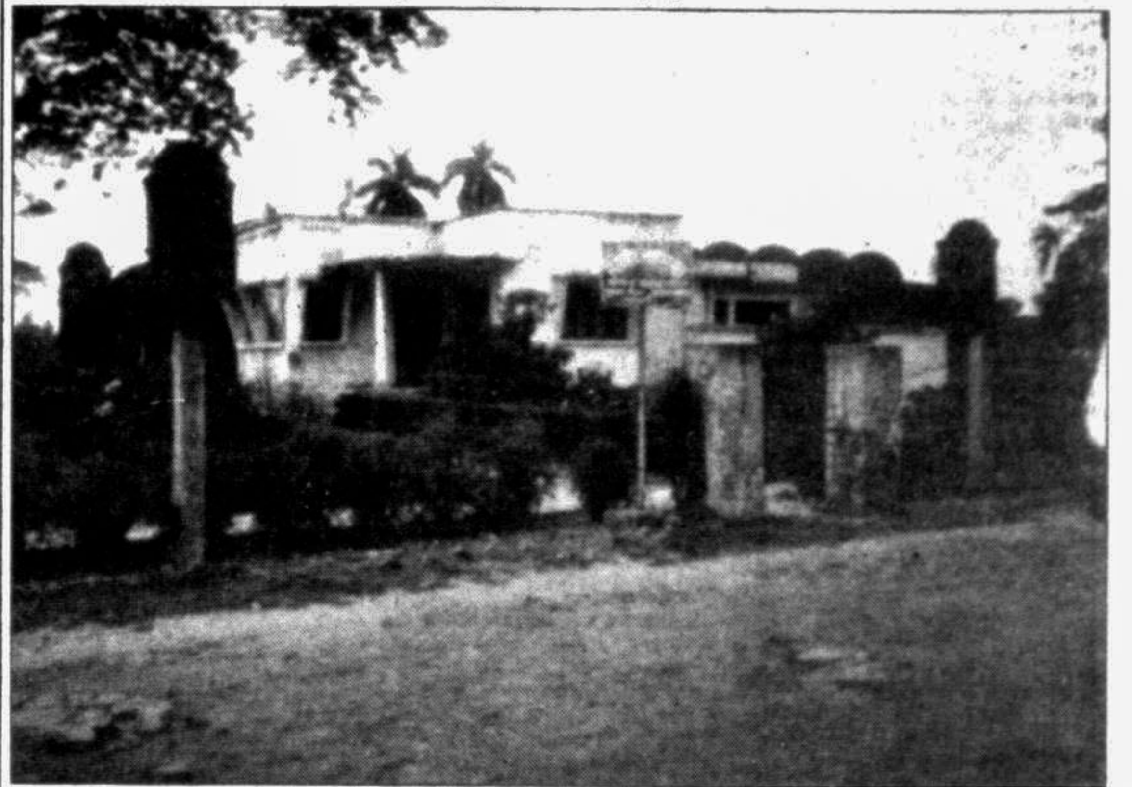
BAGERHAT: Divisional Rest House of the Directorate of Archaeology has been constructed within the compound of Shat-Goombaz. —Star photo
