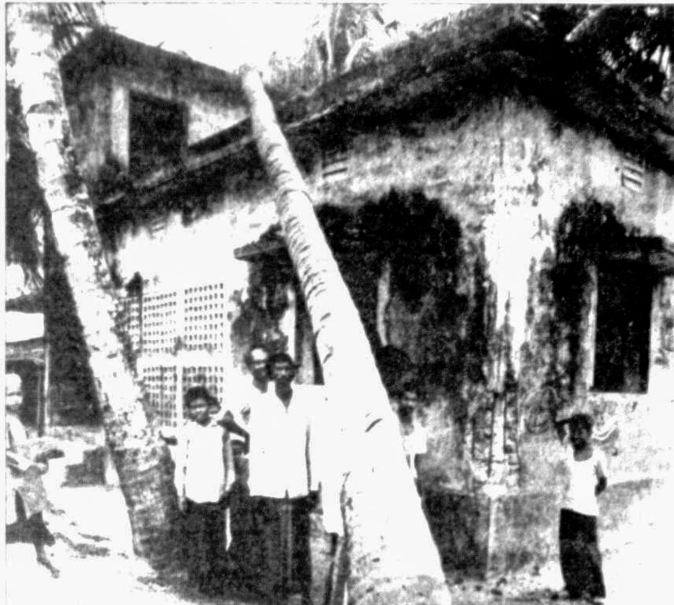
Dailapara sub-centre which was supposed to act as a shelter but nearly got swept away.
