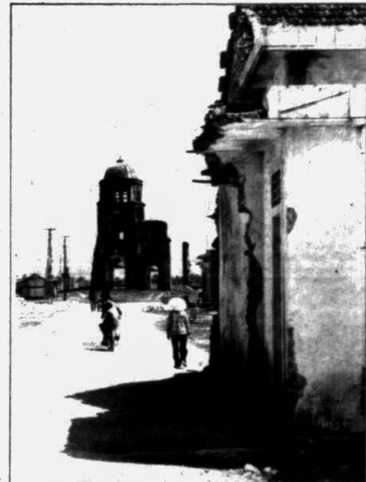
A bombed-out street in the port of Vinh in northern Vietnam. In the background is all that is left of the once imposing Catholic cathedral.
