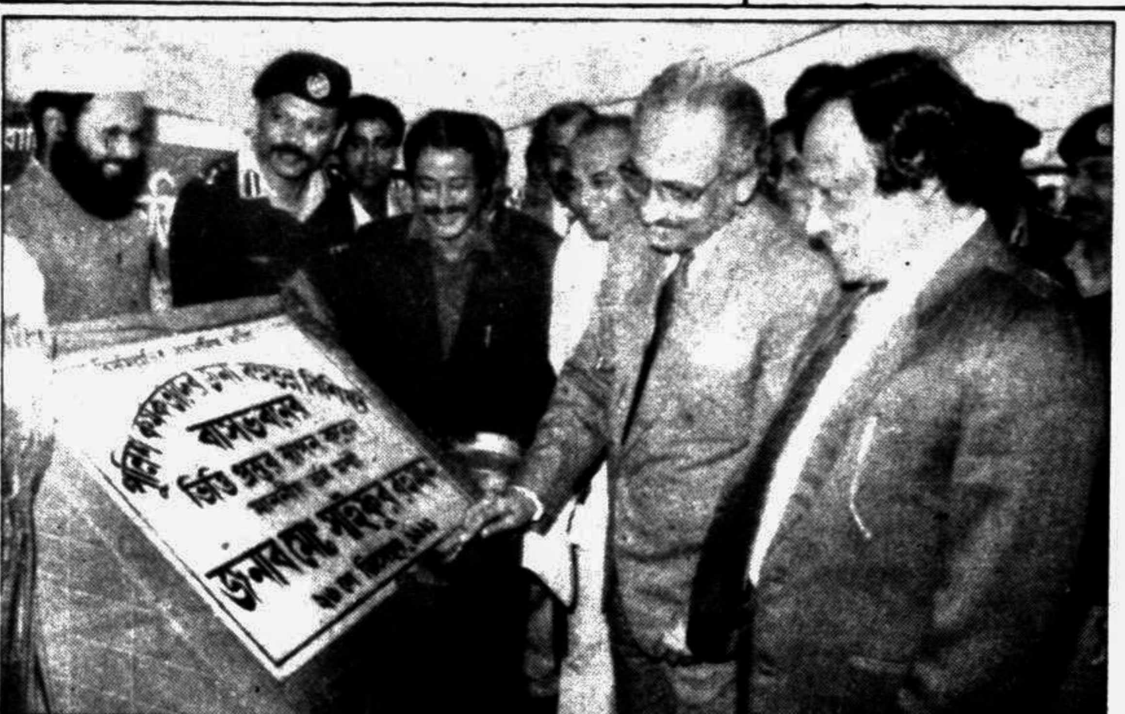
Finance Minister M Saifur Rahman Thursday laying the foundation stone of a multi-storied accommodation for police officers at Baily Square in City. —PID photo
