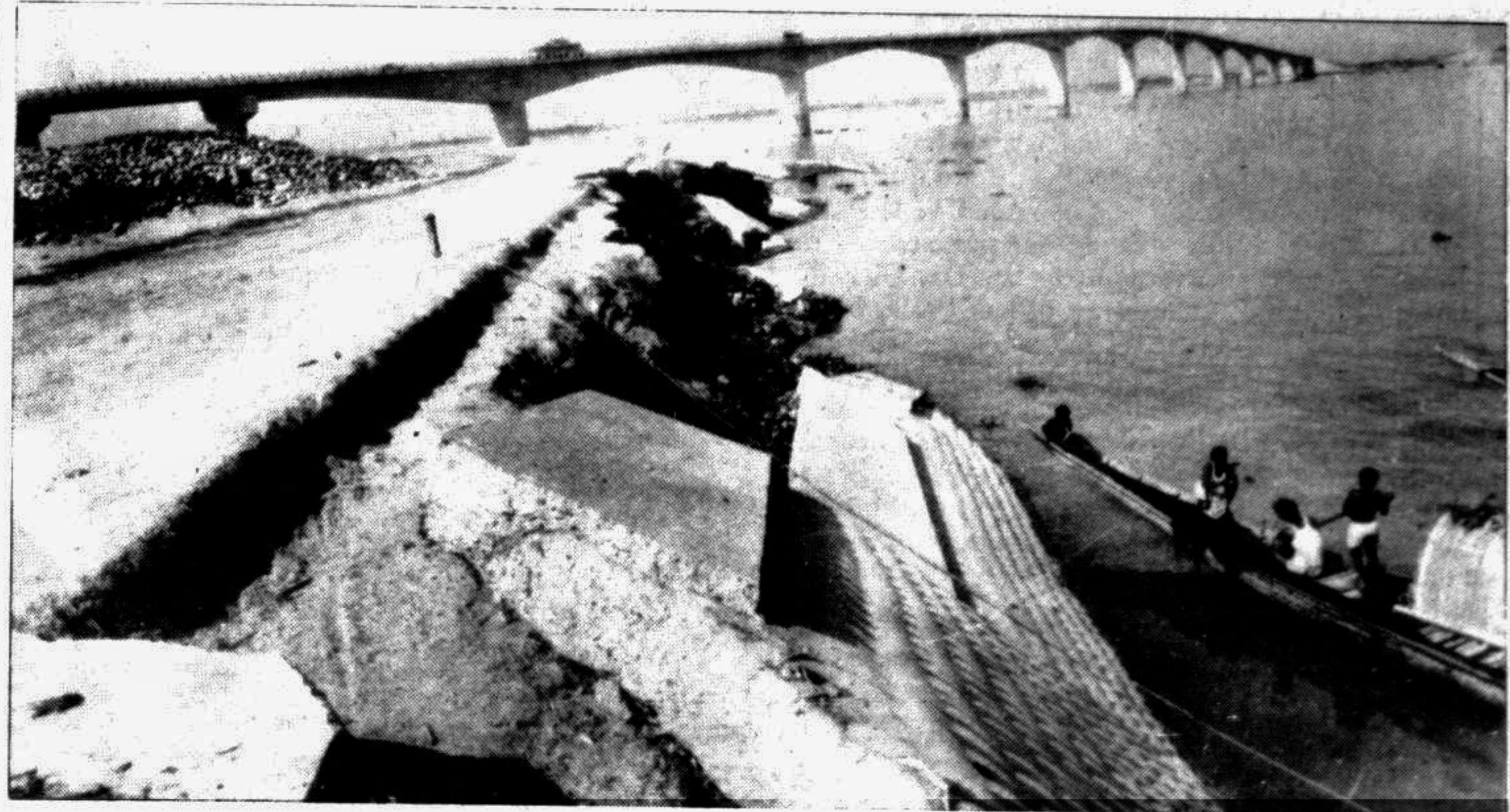
Part of the Meghna Bridge protection embankment has collapsed recently.
