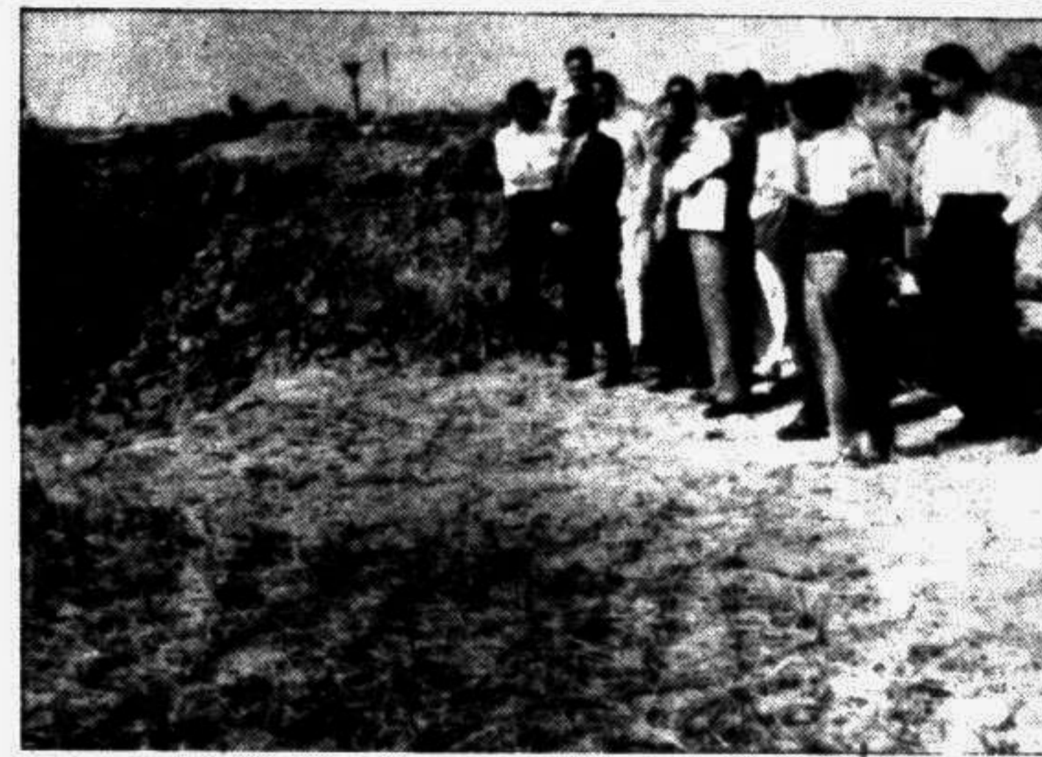
Works Minister Barrister Rafiqul Islam Mia inspecting the development work of the extended housing project of Rajuk at Uttara on Thursday. —PID photo
