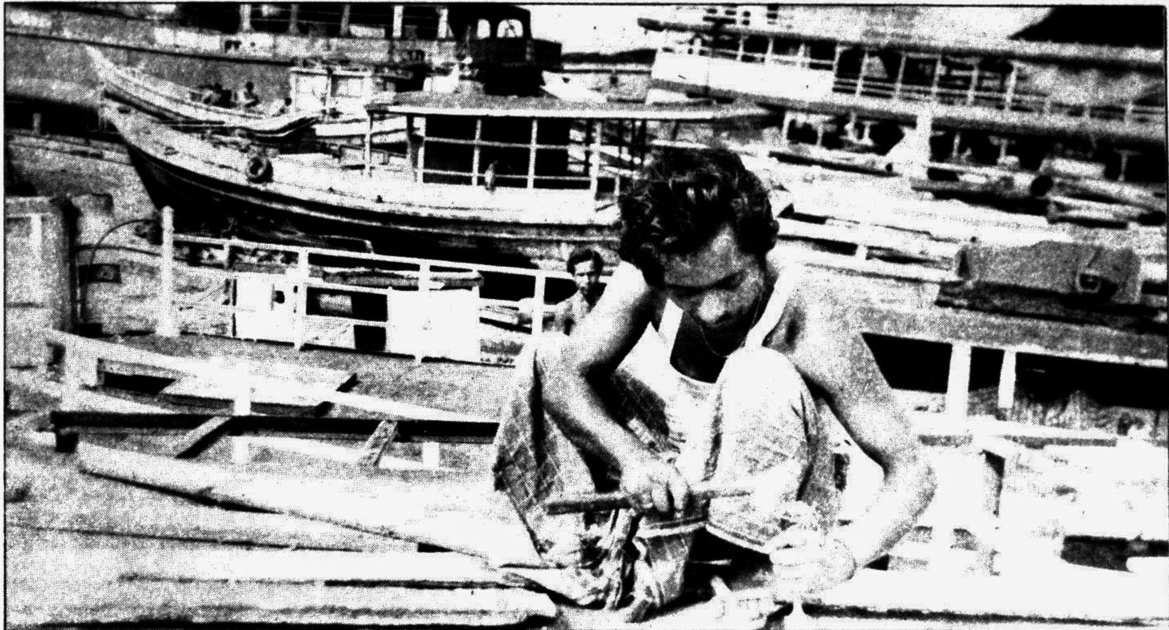
Bangladesh is a riverine country. Thousands of launches and mechanised boats ply on the river routes carrying people and merchandise round the year. Photo shows a carpenter repairing a launch at Narayanonj launch terminal. — Star photo
