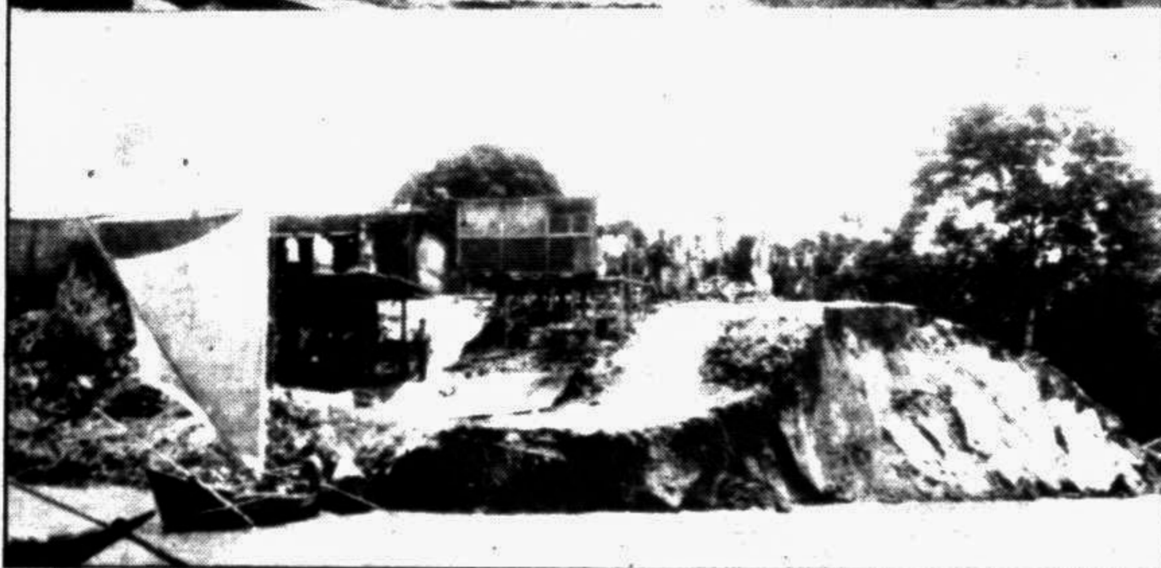
CHANDPUR: Havoc caused by the Meghna erosion. Photo shows two-storied girls high school building at Purn Bazar (top), Chandpur railway station at Natun Bazar (middle) and part of kutch bazar (bottom). —Star photo
