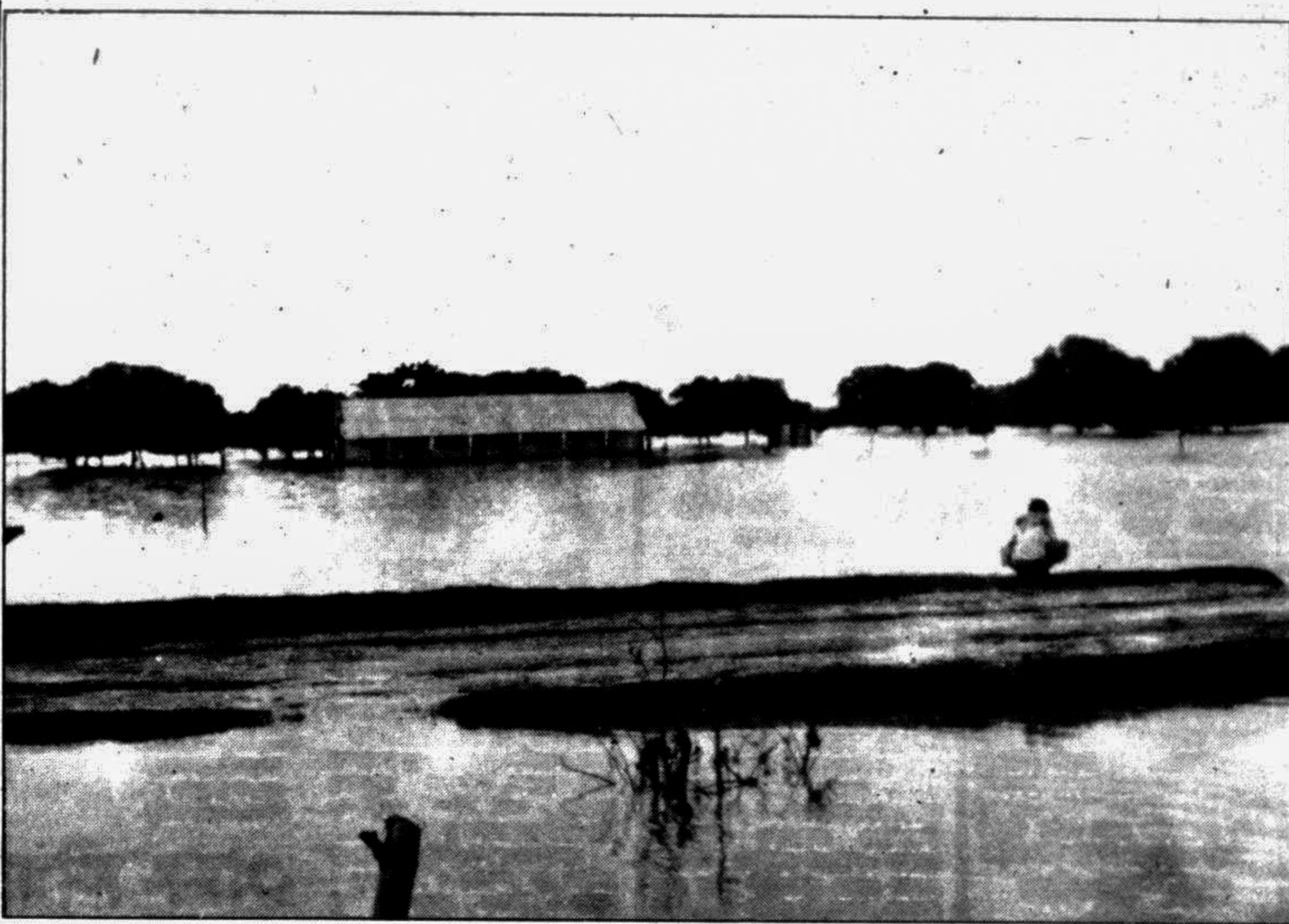
CHAPAINAWABGANJ : Narayanpur Junior High School submerged by flood water
